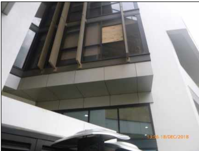
Photograph 3 – Cladding panels identify on the facade on the northern elevation of the building.
