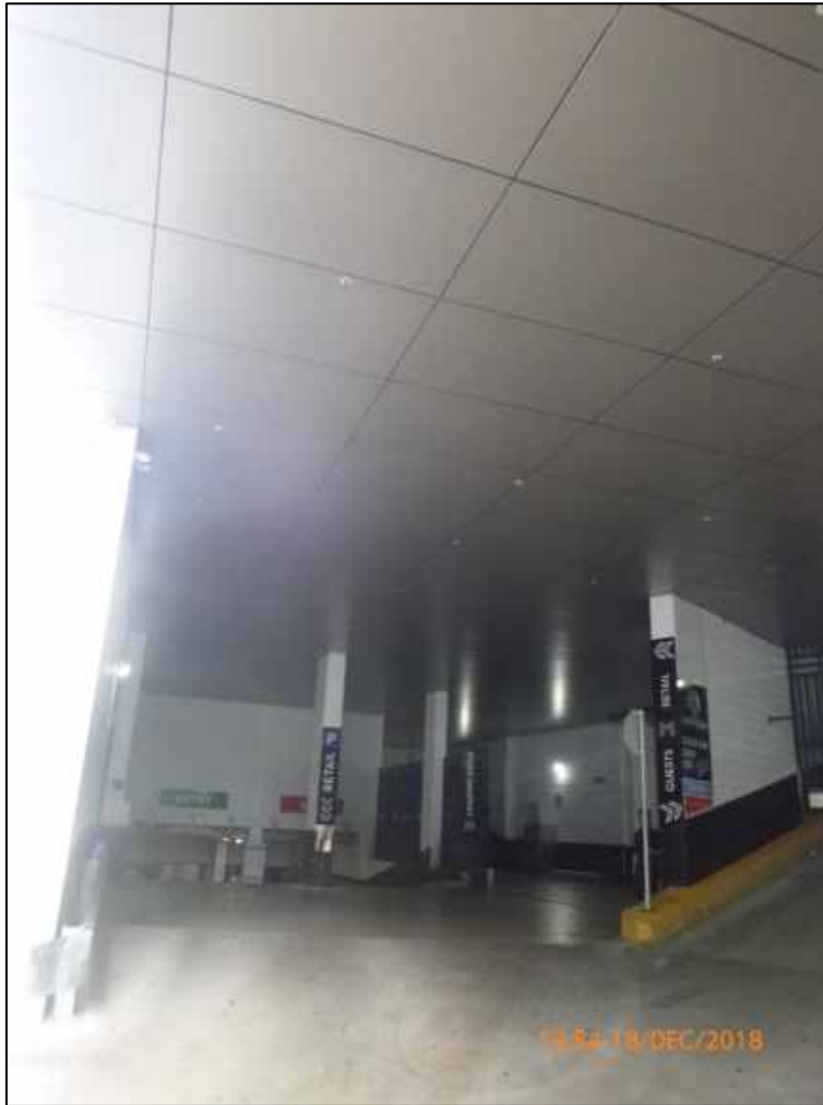
Photograph 2 – Cladding panels identify on the soffit of the carpark entrance on the eastern elevation.
