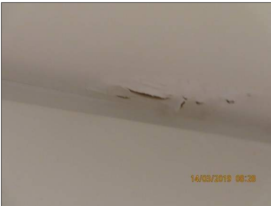
Photograph 11: Showing blistering plasterboard to access hatch in the Kitchen of Unit 8.
