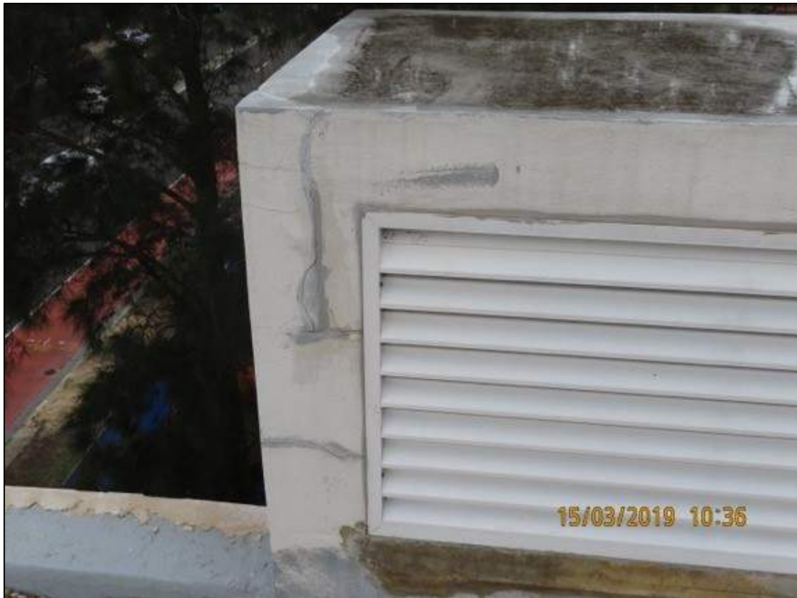
Photograph 72: Showing evidence of previous patch repairs to rooftop façade wall.
