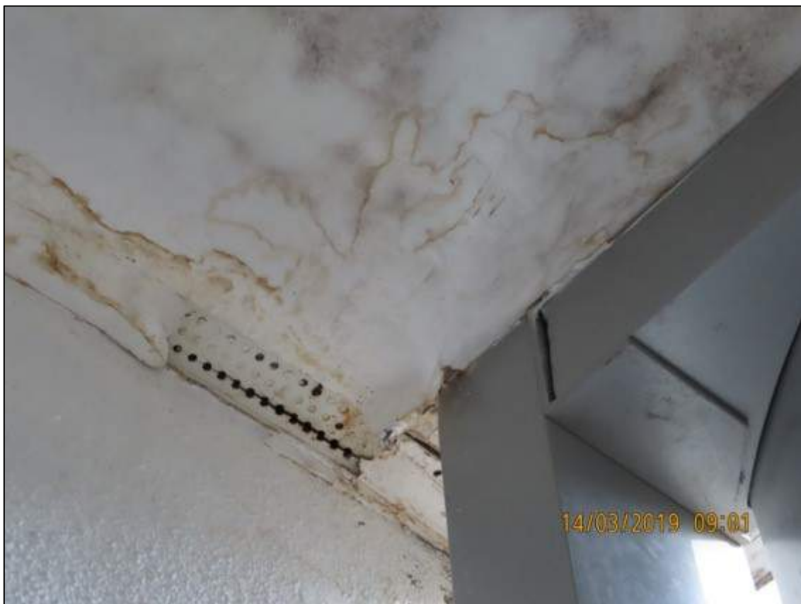
Photograph 49: Showing further view of water damage to plasterboard ceiling opposite to Unit 14.
