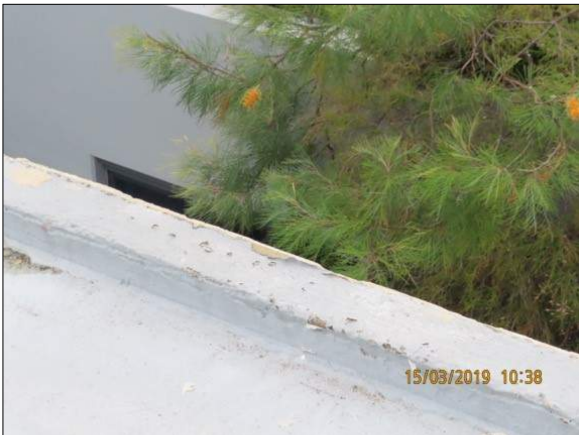
Photograph 77: Showing blistering membrane to perimeter edge of rooftop.
