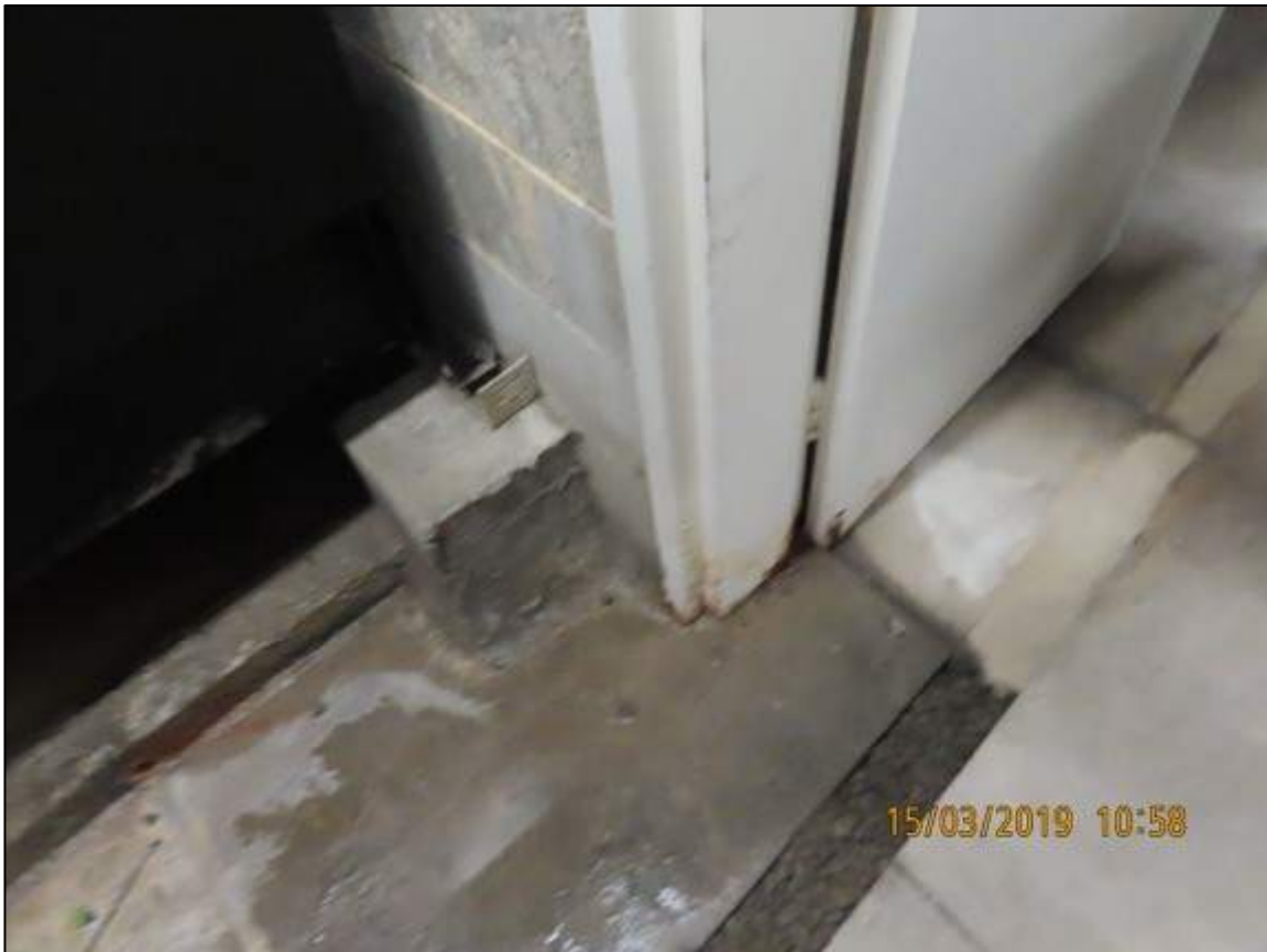
Photograph 62: Showing corrosion to door jambs of Car Motor Lift Room on Level 3 basement.
