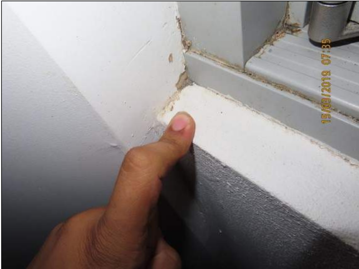
Photograph 38: Showing water damage and staining adjacent to Bedroom window of Unit 20.
