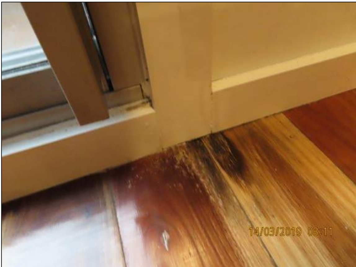
Photograph 7: Showing consequential damages in form of water damage to timber floorboards of Living Room in Unit 5.
