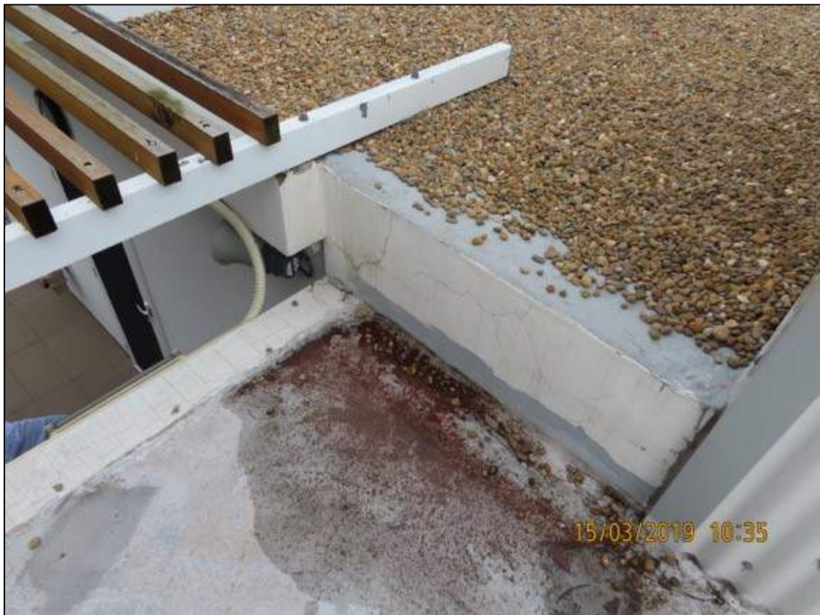
Photograph 69: Showing ponding water adjacent to ballast rooftop.
