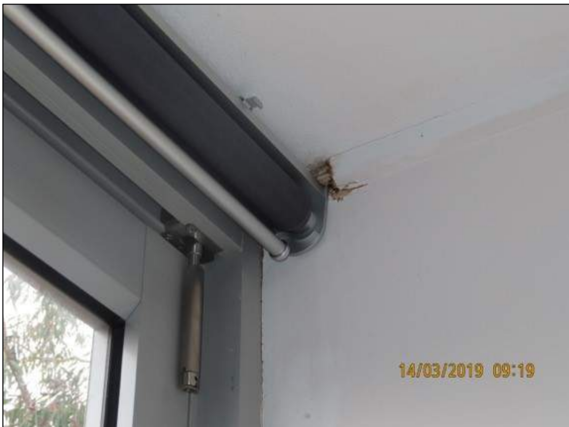
Photograph 21: Showing water damage to ceiling lining adjacent to head of Enclosed Balcony windows of Unit 15.
