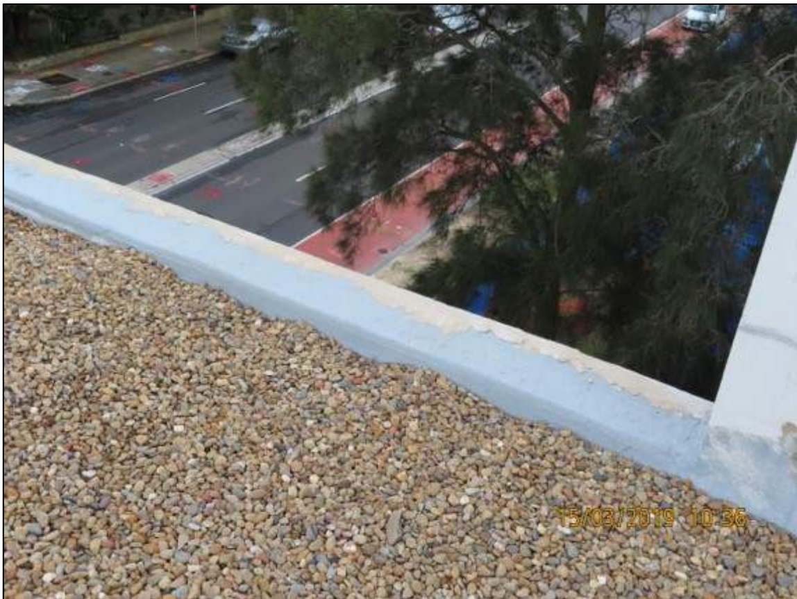
Photograph 73: Showing delamination of waterproofing membrane to perimeter edge.
