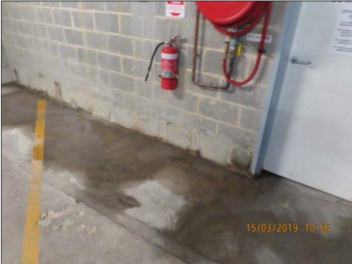
Photograph 60: Showing further view of water ponding adjacent to northern fire stairs on Level 3 basement.
