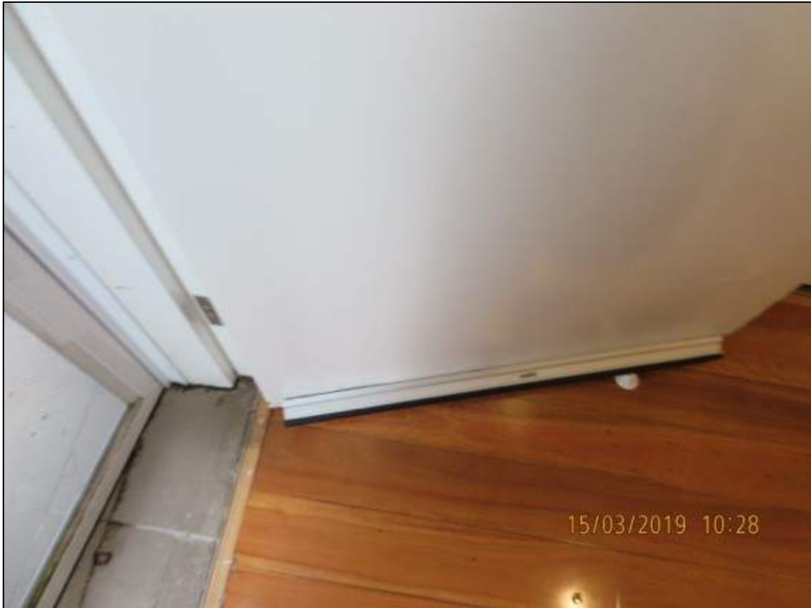
Photograph 40: Showing water damage to entry door of Unit 22.
