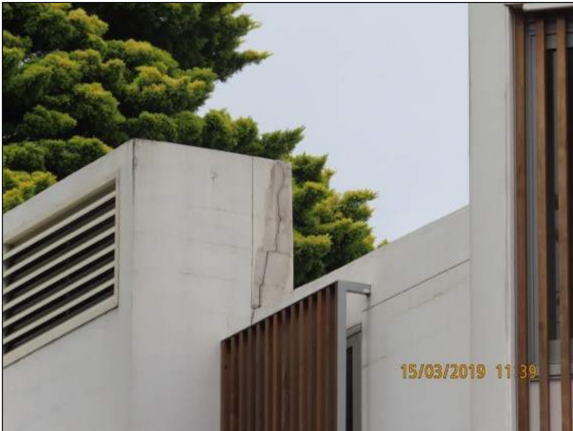
Photograph 66: Showing stepped cracking to eastern rooftop wall.
