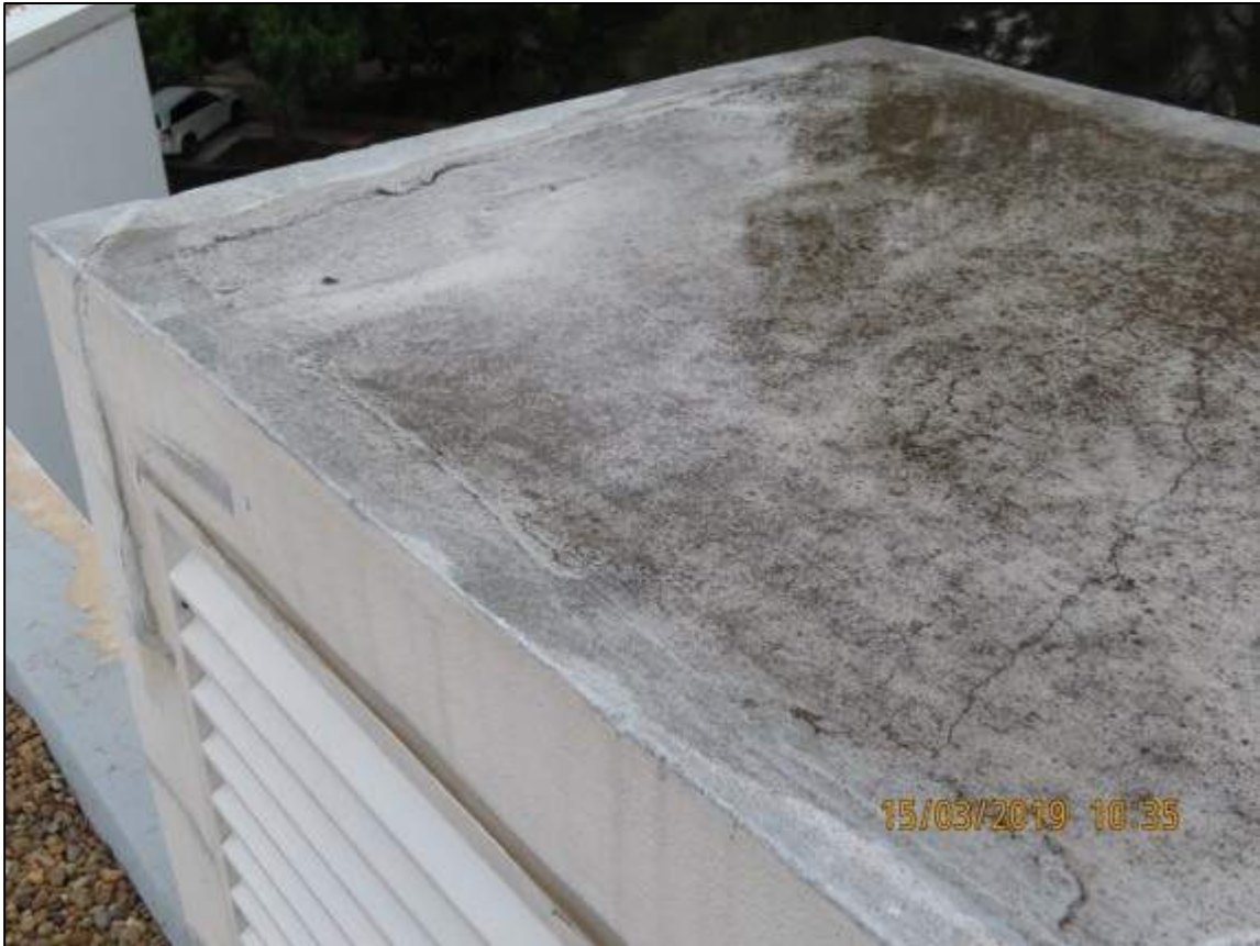
Photograph 70: Showing ponding water to exposed area of rooftop.
