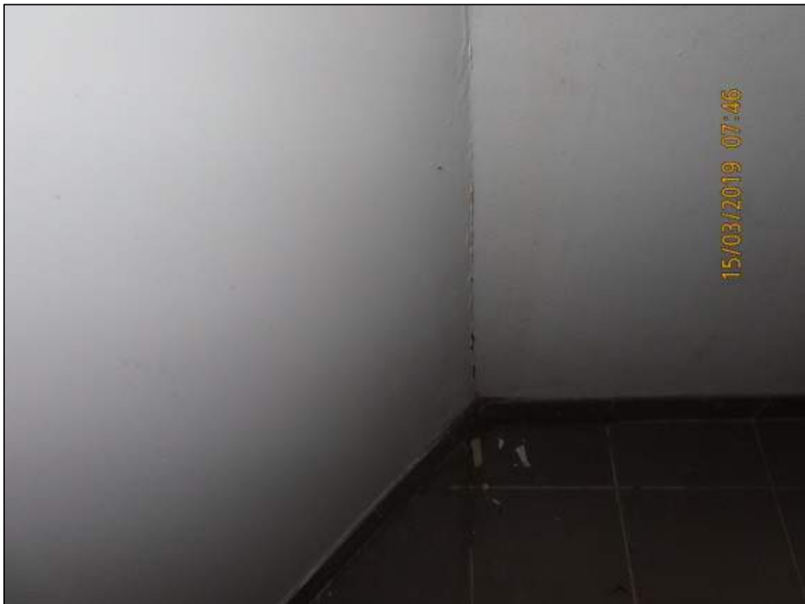
Photograph 27: Showing blistering plasterboard below Enclosed Balcony windows of Unit 18.
