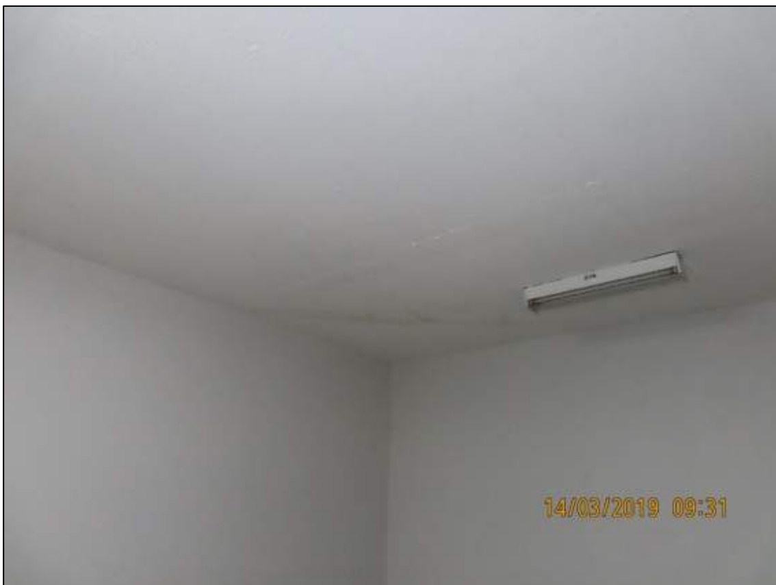
Photograph 53: Showing further view of water staining to soffit of Level 3 southern fire stairs.
