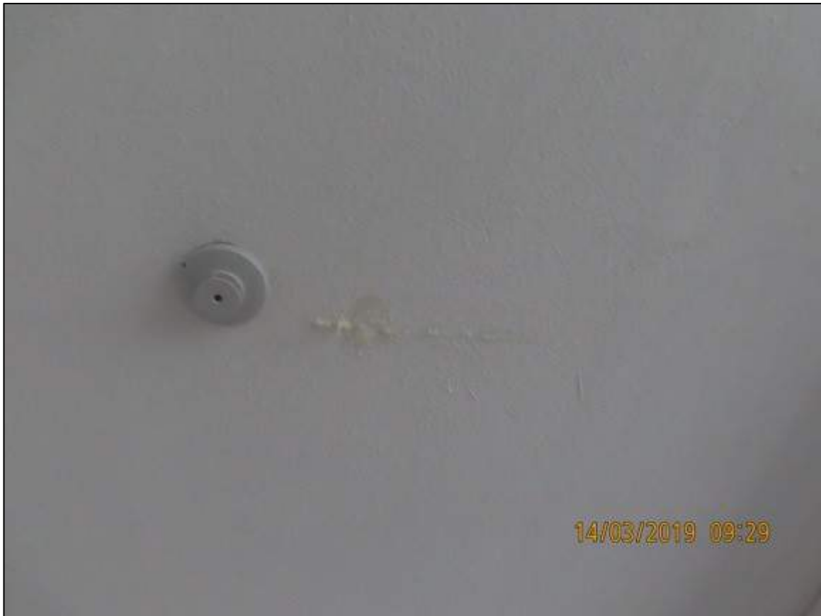
Photograph 46: Showing efflorescence leaching out of cracking to soffit of Level 2 internal common area between Units 15 and 16.
