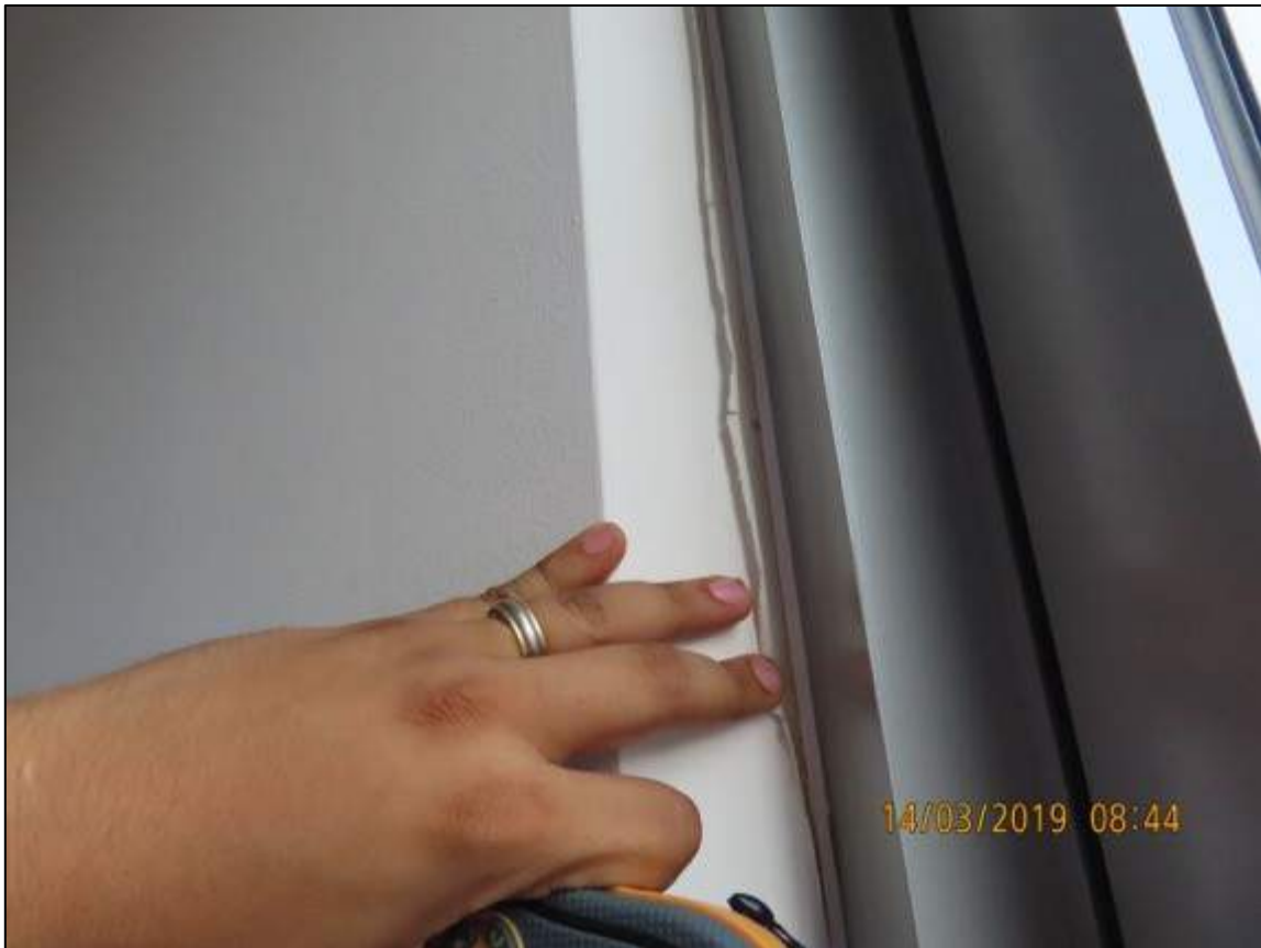
Photograph 18: Showing delamination of plasterboard adjacent to Enclosed balcony window of Unit 13.
