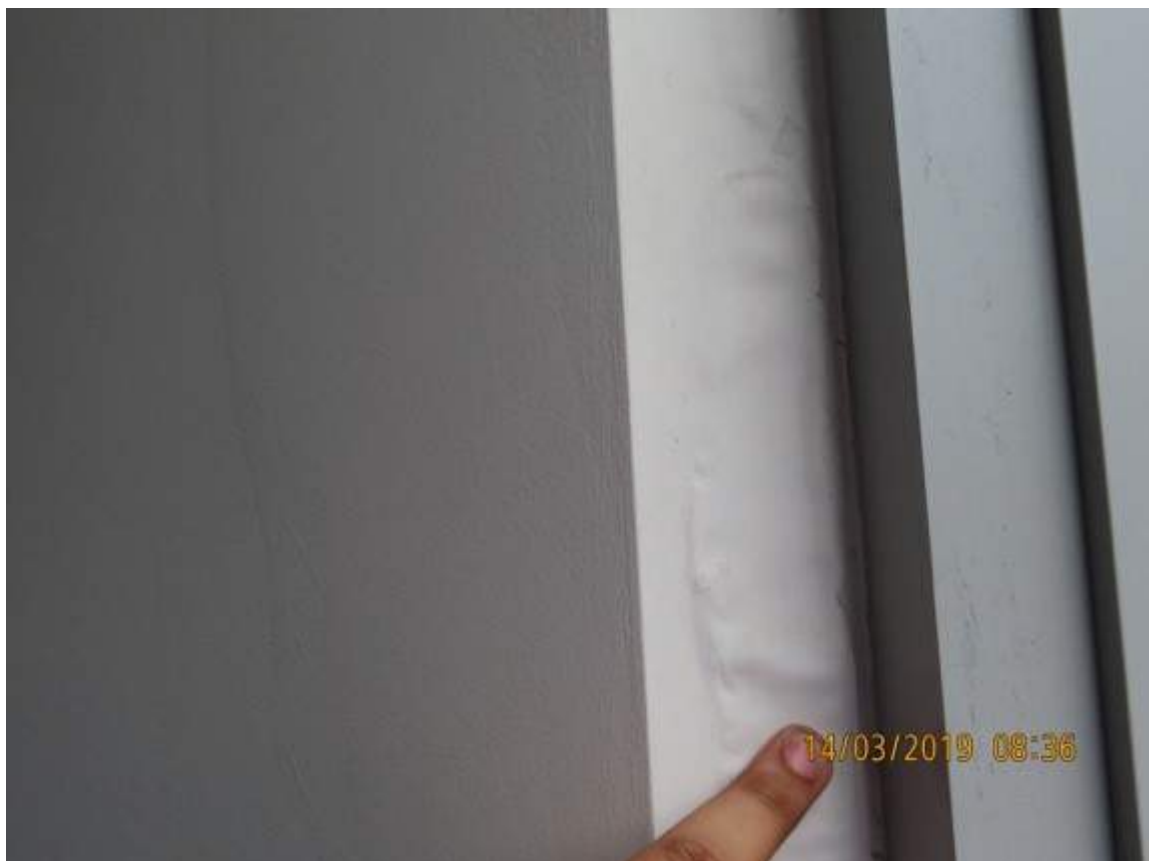
Photograph 17: Showing blistering plasterboard adjacent to Enclosed balcony windows of Unit 11.
