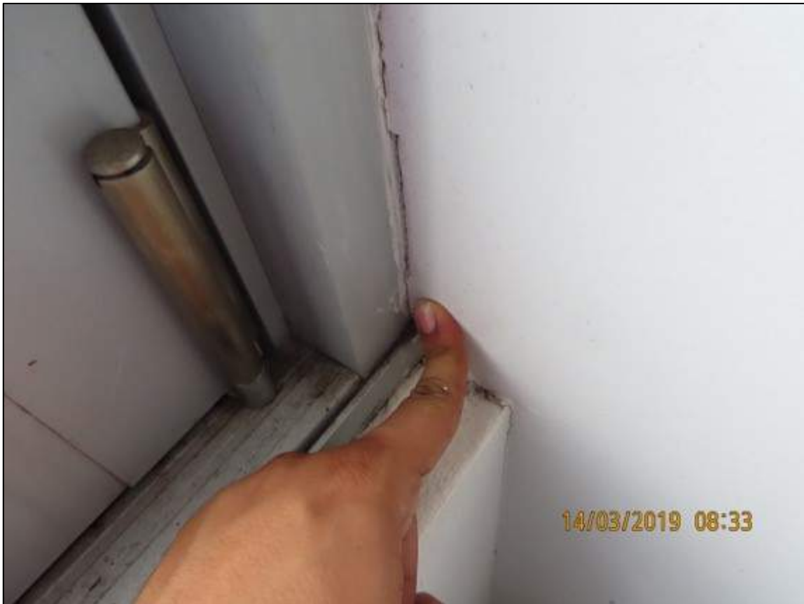
Photograph 14: Showing water damage adjacent to Enclosed balcony windows of Unit 10.
