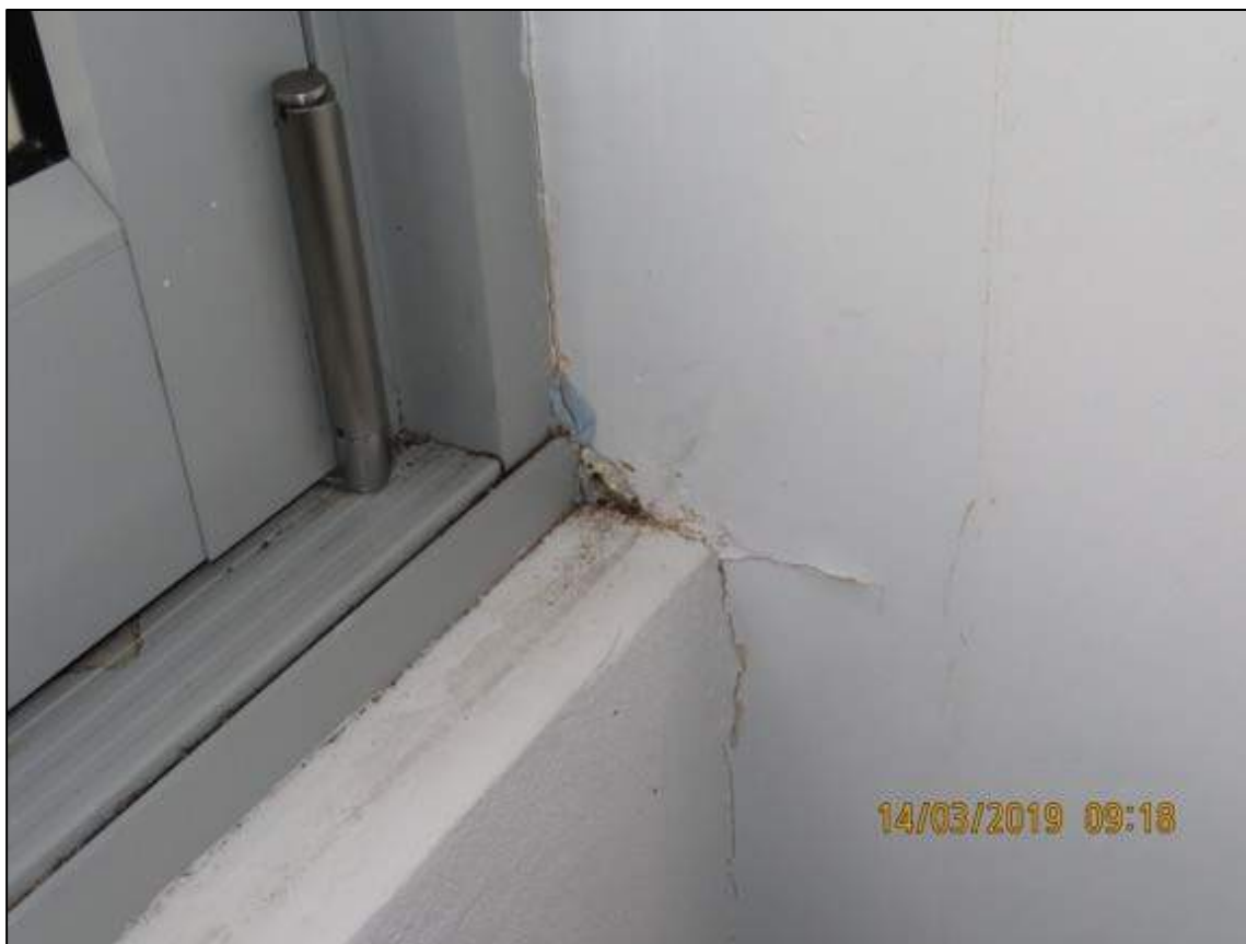
Photograph 22: Showing water damage adjacent to base of Enclosed Balcony windows of Unit 15.
