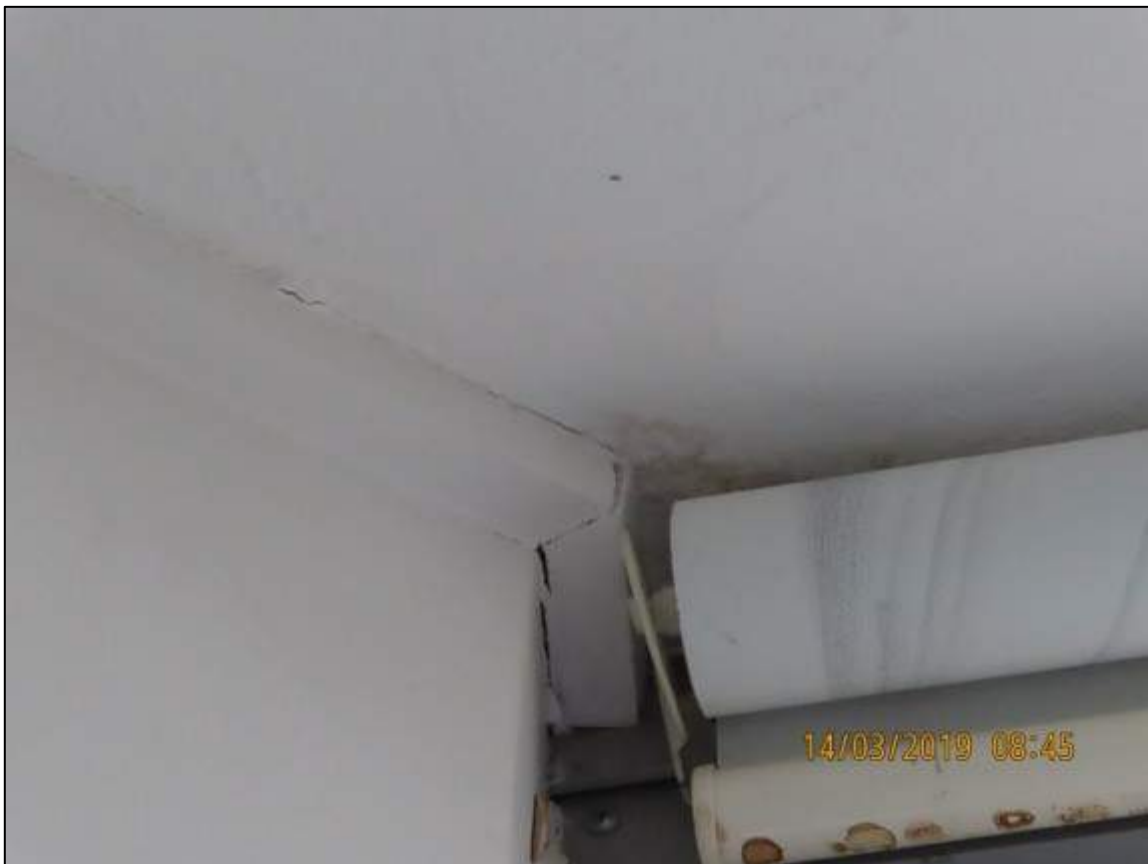
Photograph 19: Showing water damage and staining to ceiling adjacent to head of Enclosed Balcony windows in Unit 13.
