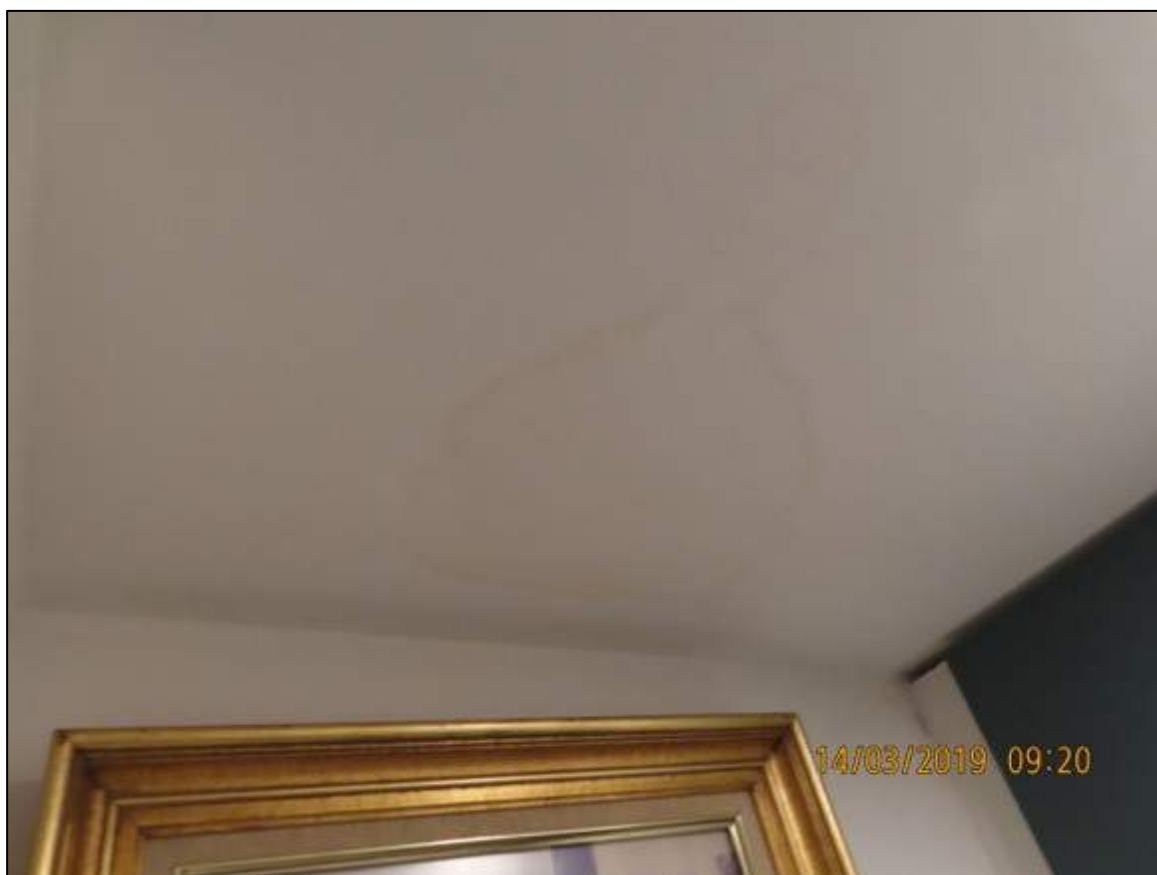
Photograph 23: Showing water staining to ceiling of Bathroom in Unit 15.
