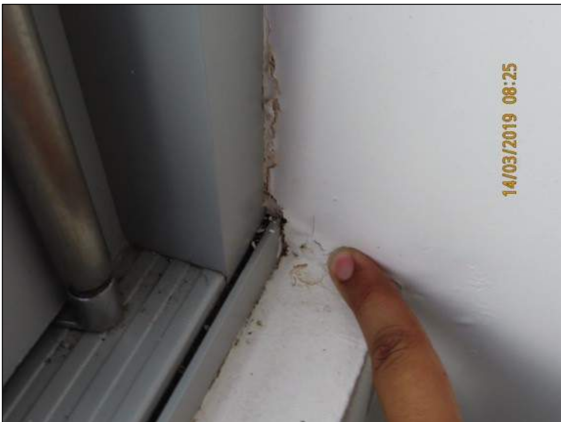
Photograph 9: Showing blistering plasterboard wall and water damage adjacent to the Enclosed balcony windows in Unit 8.
