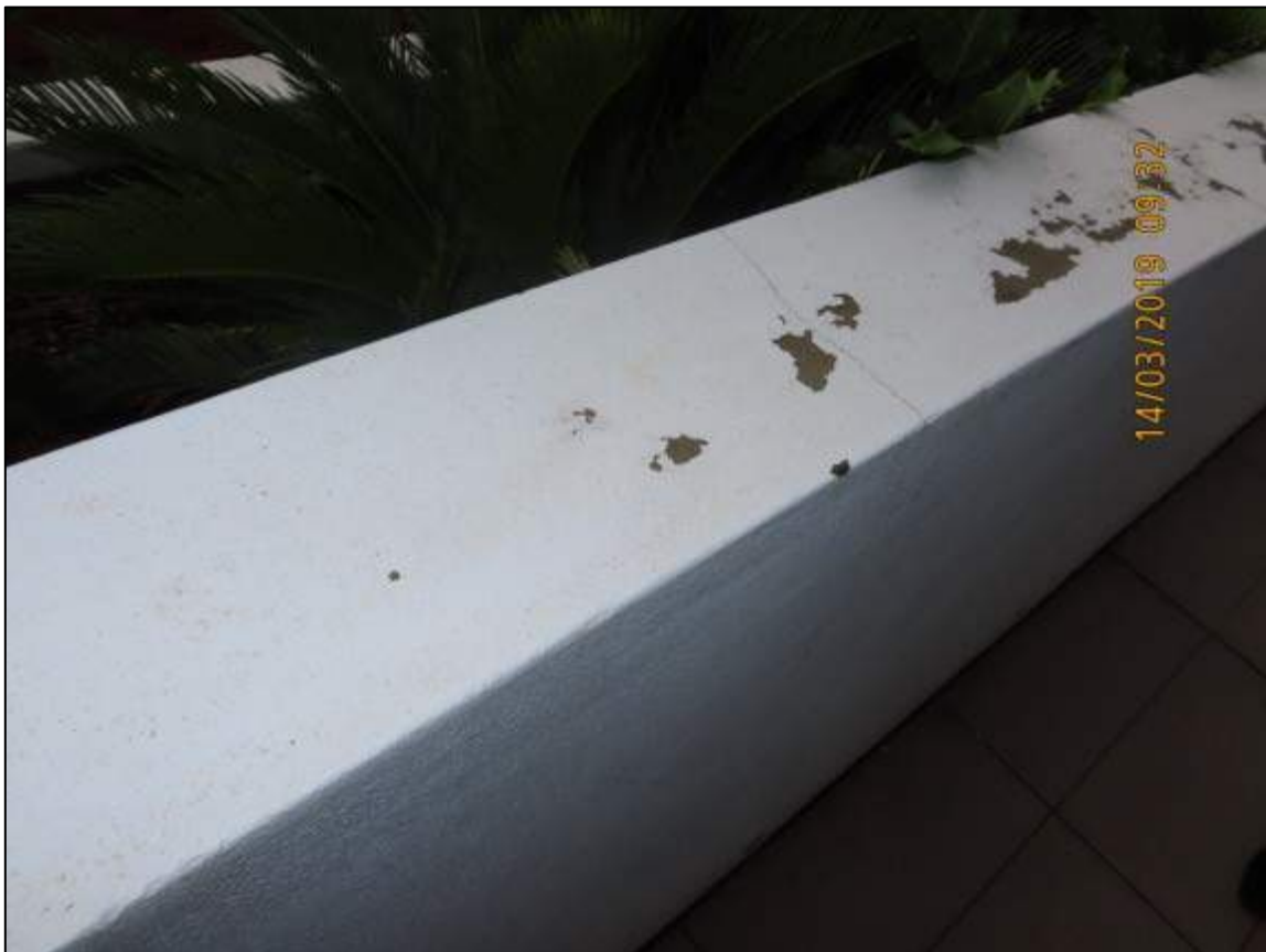
Photograph 55: Showing cracking and delamination to paint system to Level 3 external common area planterboxes.
