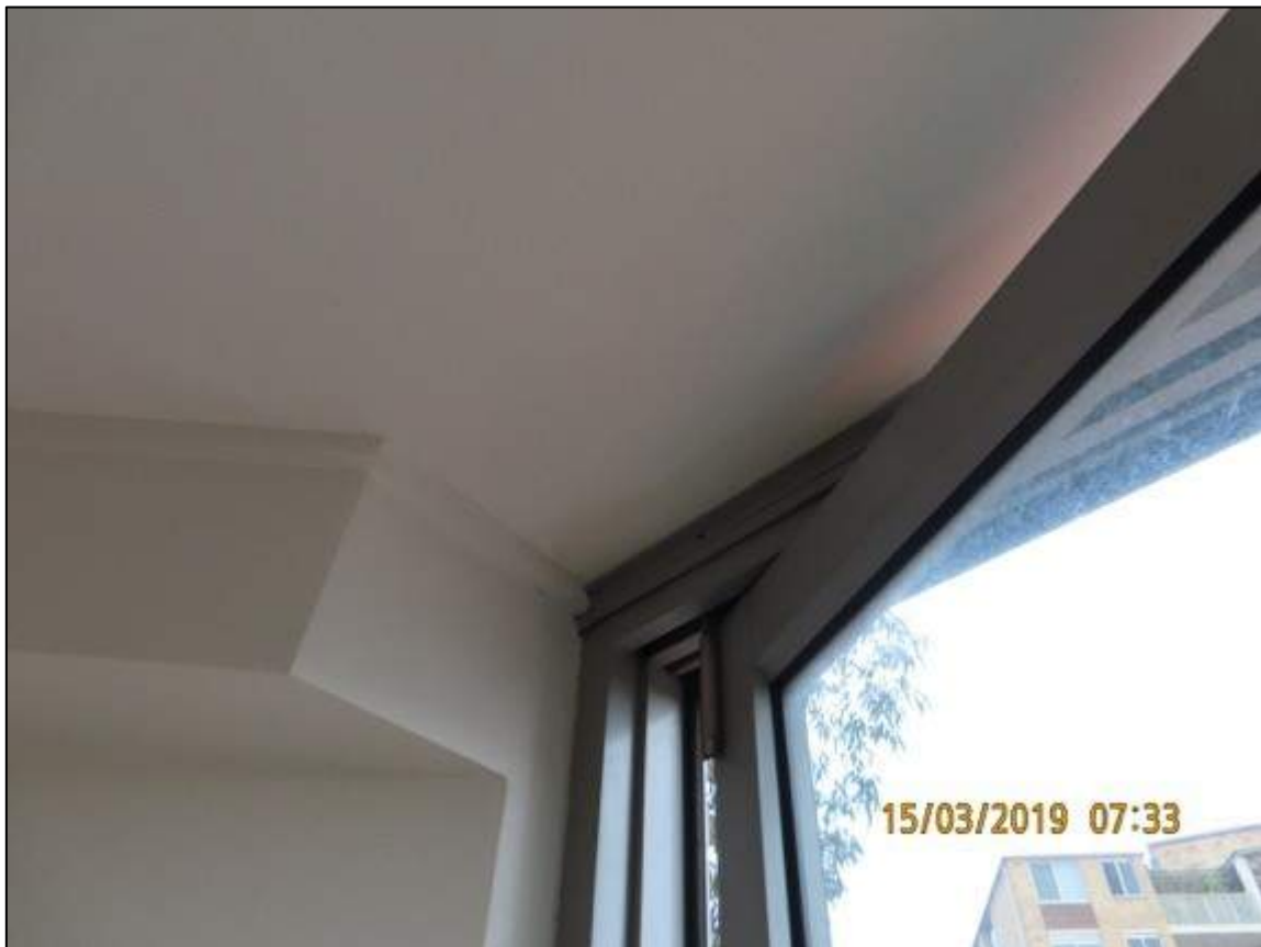
Photograph 25: Showing water staining adjacent to head of Enclosed Balcony windows of Unit 17.
