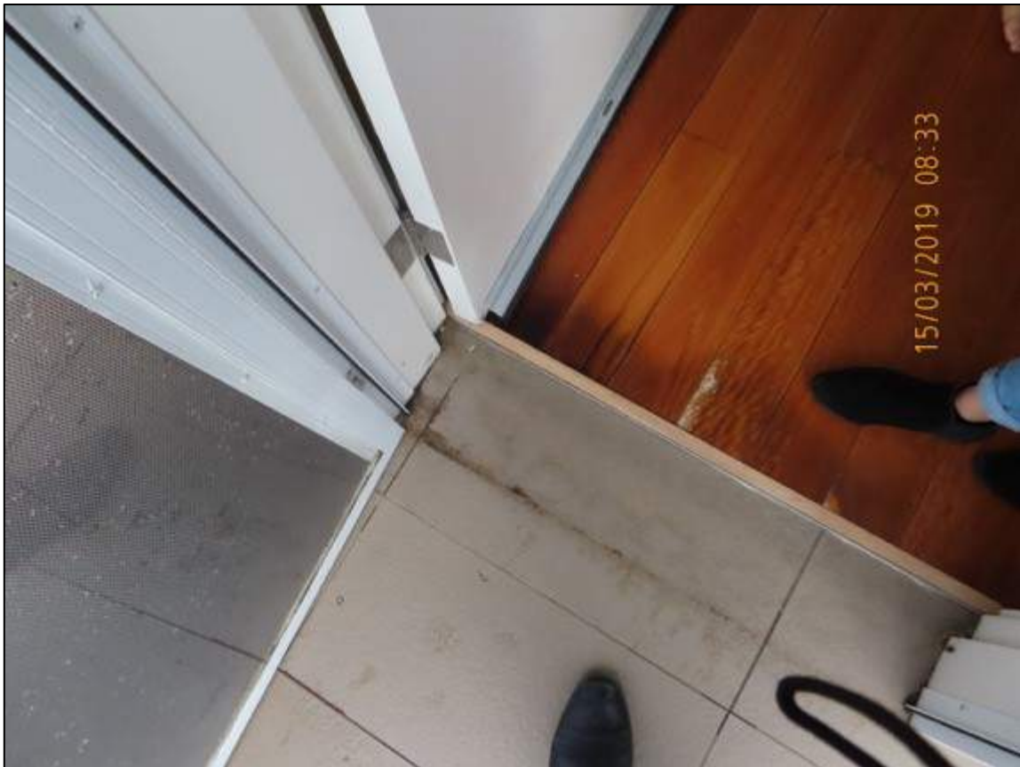
Photograph 42: Showing water damage and staining to timber floorboard adjacent to entry door of Unit 26.
