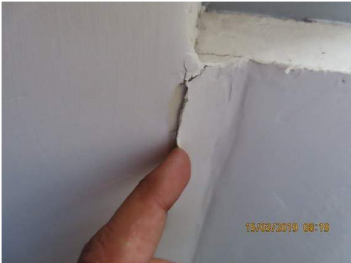
Photograph 44: Showing delaminating plasterboard below Enclosed Balcony windows of Unit 28.
