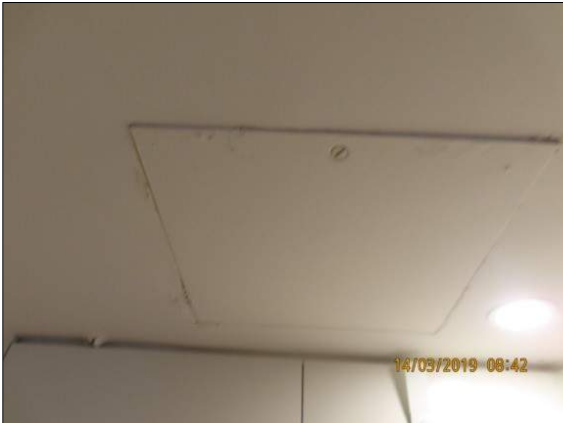
Photograph 20: Showing blistering paint to access hatch in Kitchen of Unit 13.
