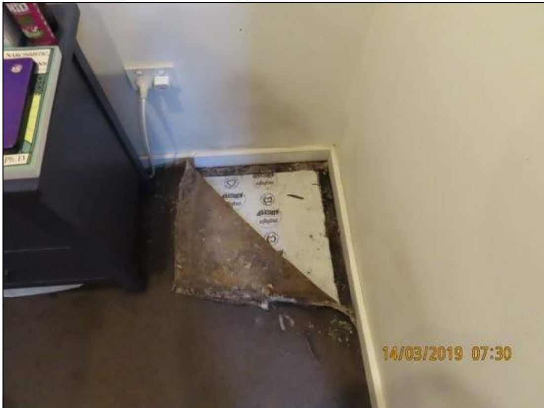
Photograph 1: Showing mould growth and water staining to smooth edge of carpet adjacent to courtyard sliding door of Bedroom 1 in Unit 4.
