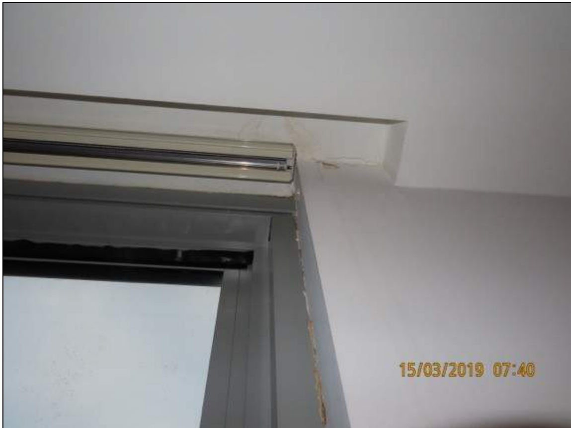
Photograph 34: Showing water damage and staining to head of Bedroom windows of Unit 19.
