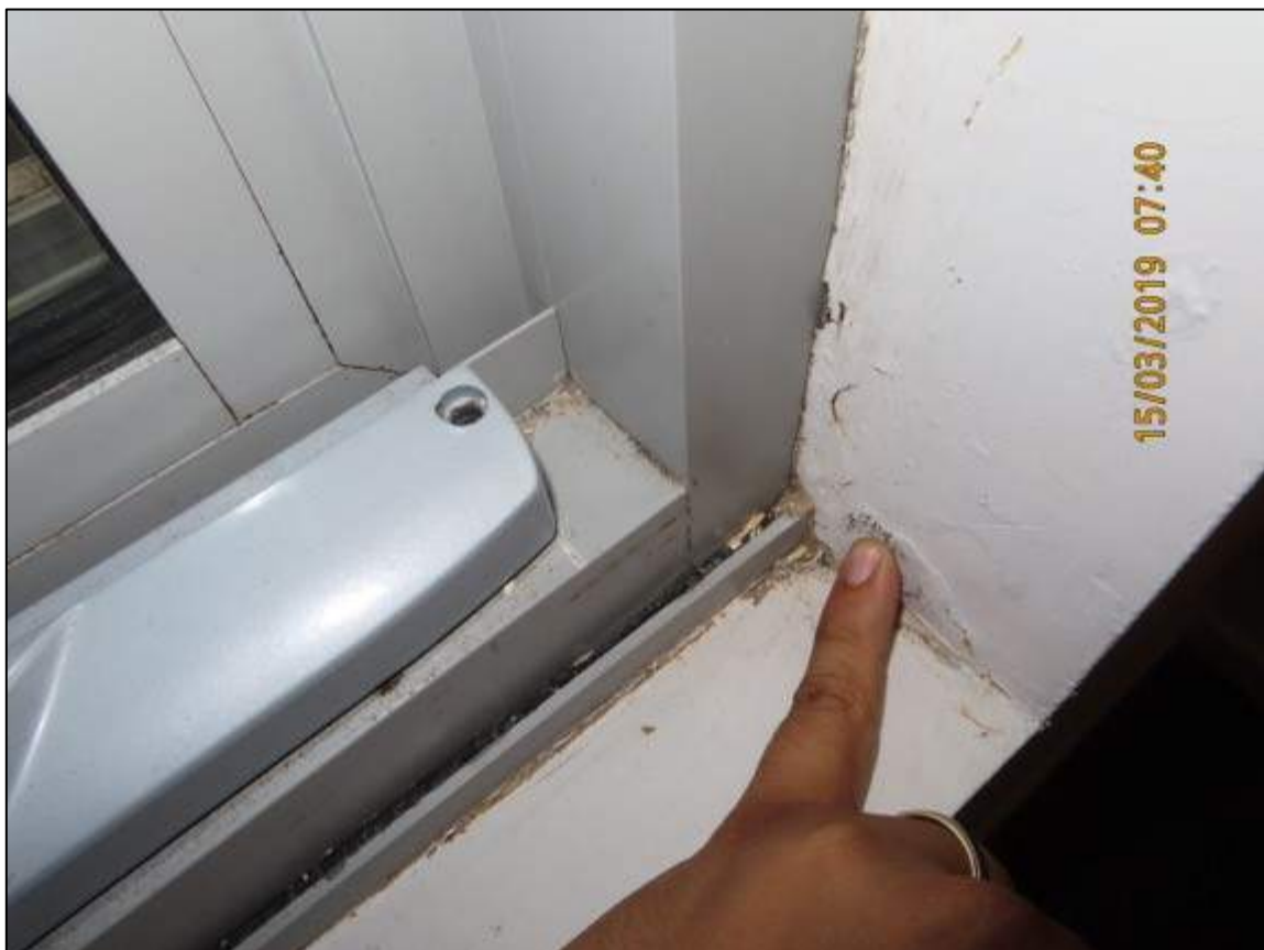
Photograph 35: Showing water damage and staining to head of Bedroom windows of Unit 19.
