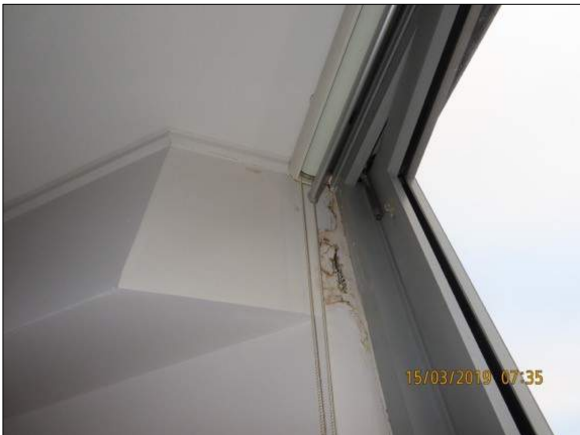
Photograph 37: Showing water damage and staining adjacent to Bedroom window of Unit 20.
