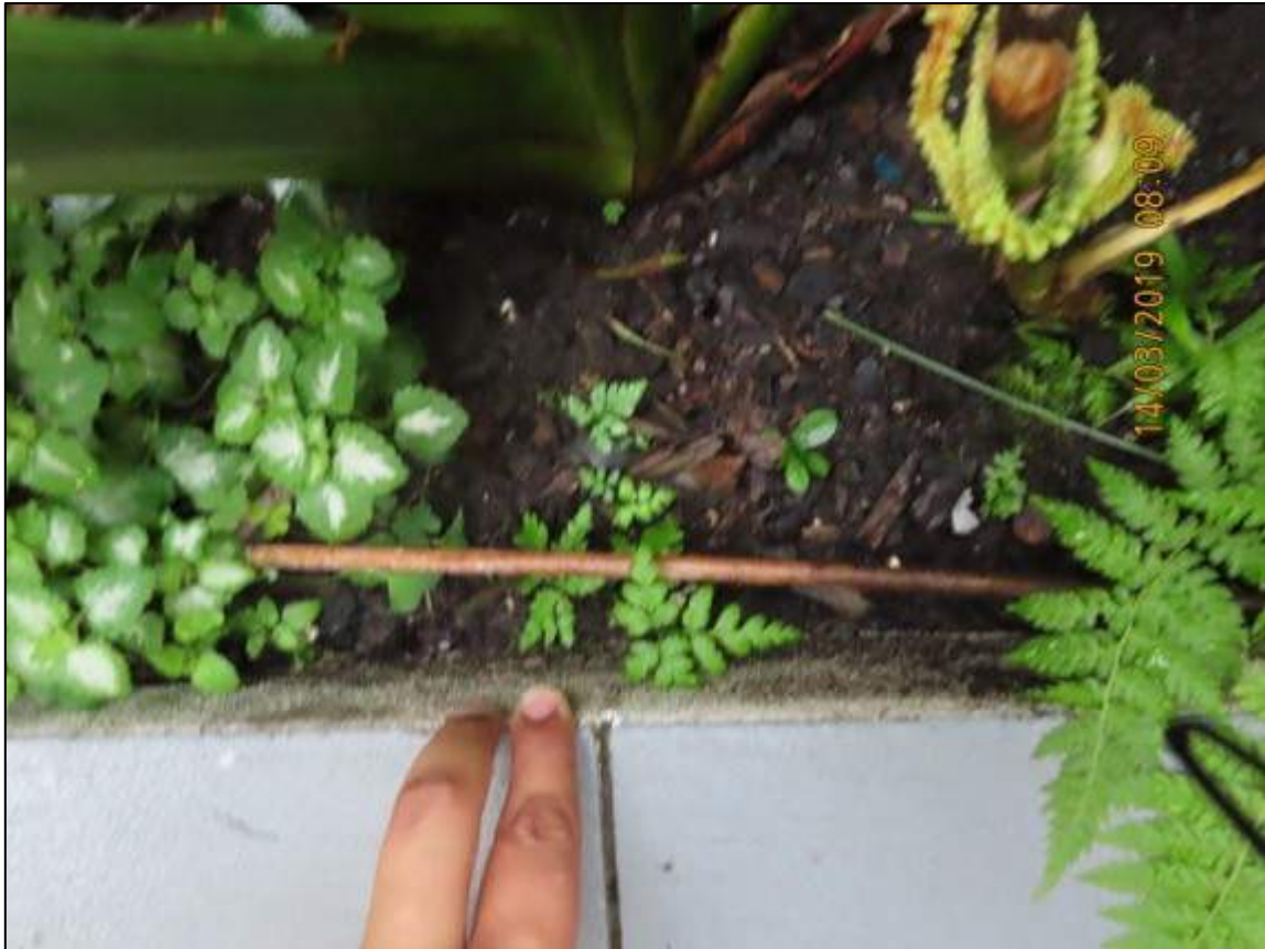
Photograph 6: Showing inadequate termination of waterproofing membrane system of courtyard planterboxes of Unit 5.
