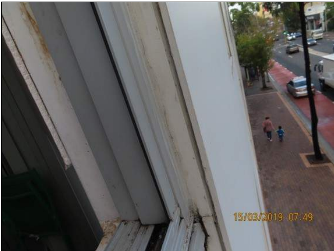
Photograph 31: Showing water staining to external facades of Enclosed Balcony windows of Unit 18.
