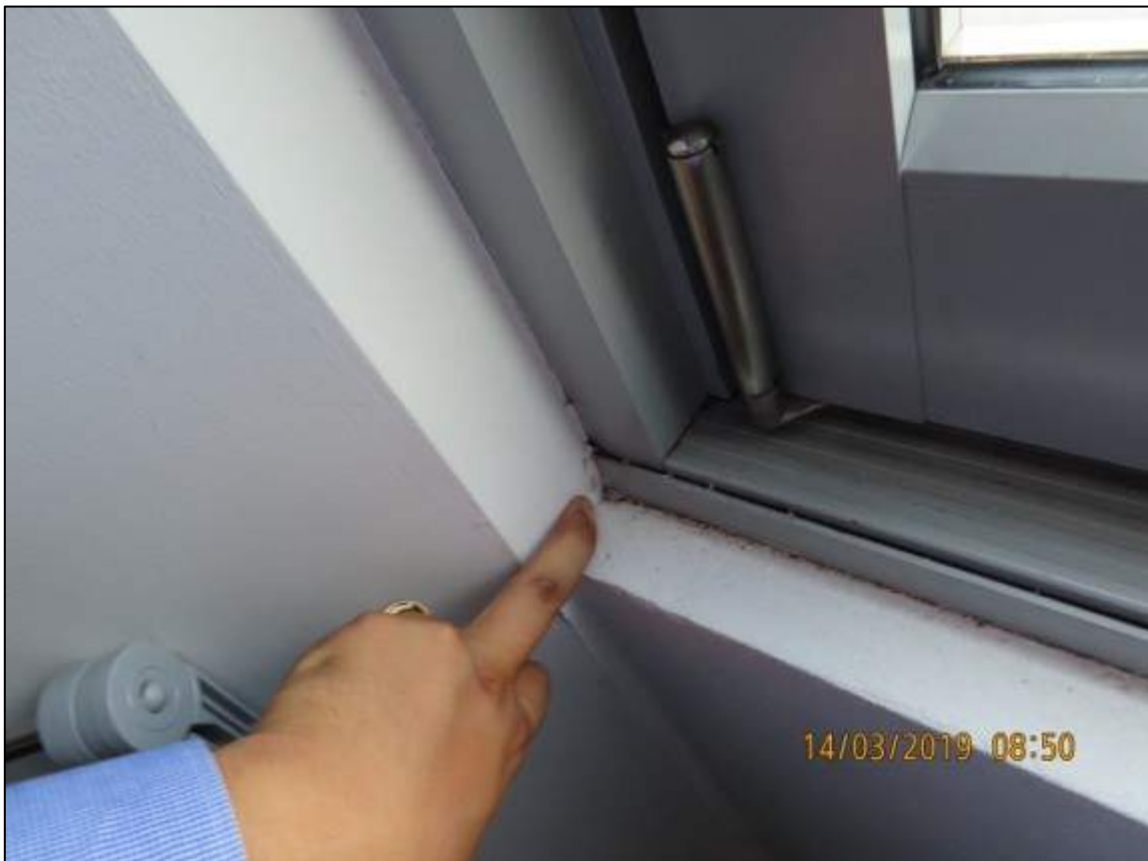
Photograph 13: Showing water damage and blistering plasterboard adjacent to Enclosed balcony window of Unit 9.
