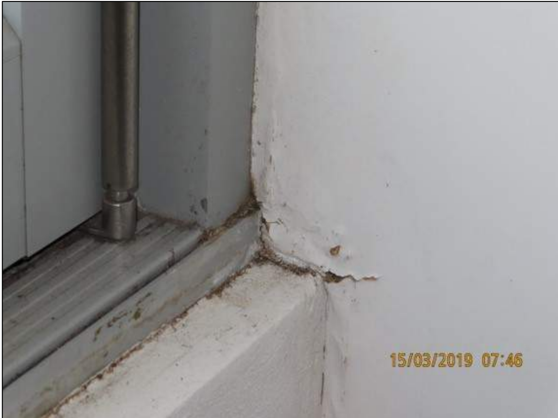
Photograph 28: Showing water damage adjacent to Enclosed Balcony windows of Unit 18.
