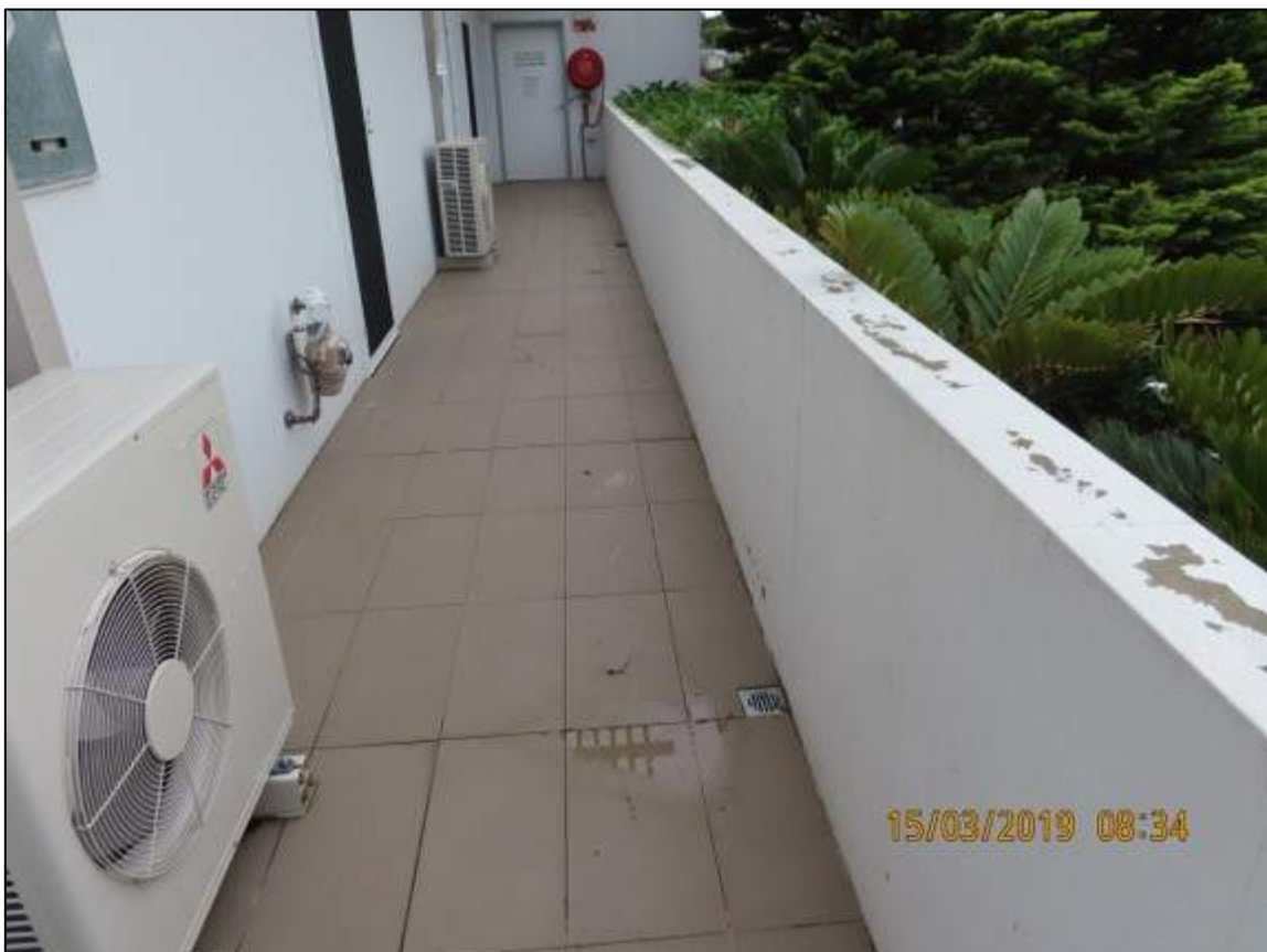
Photograph 43: Showing blockage to drainage outlet opposite Unit 26.
