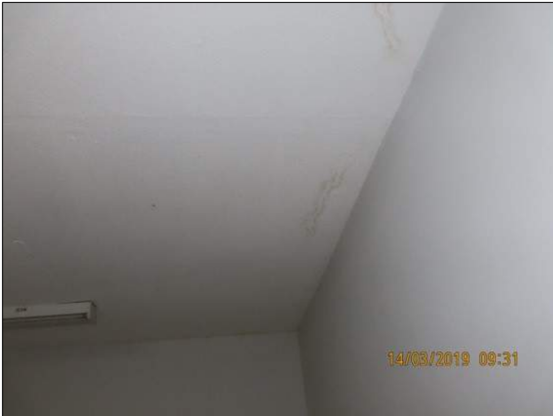
Photograph 52: Showing water staining to soffit of Level 3 southern fire stairs.
