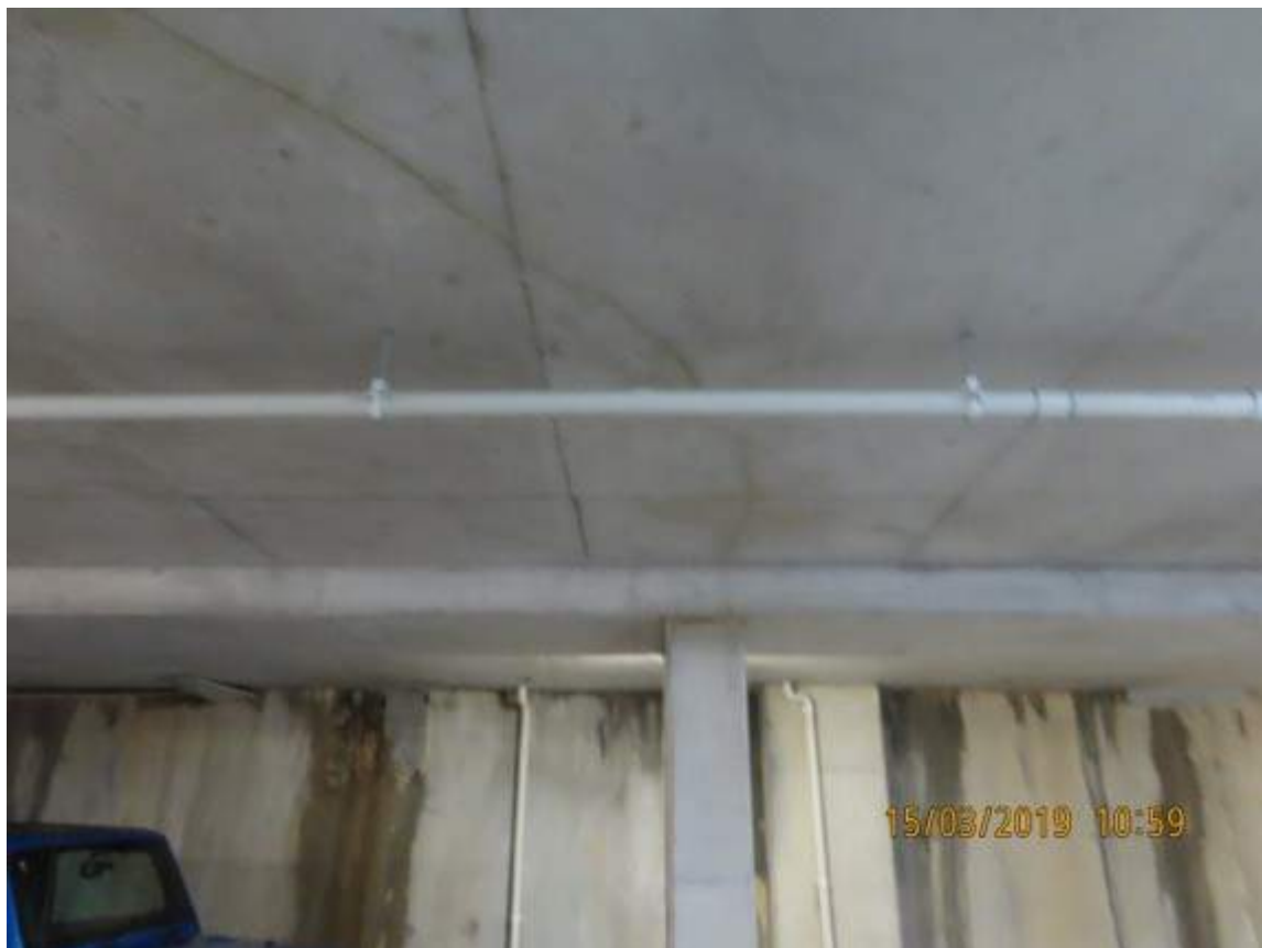
Photograph 63: Showing efflorescence emanating from cracking to soffit above car spaces 27 and 28.
