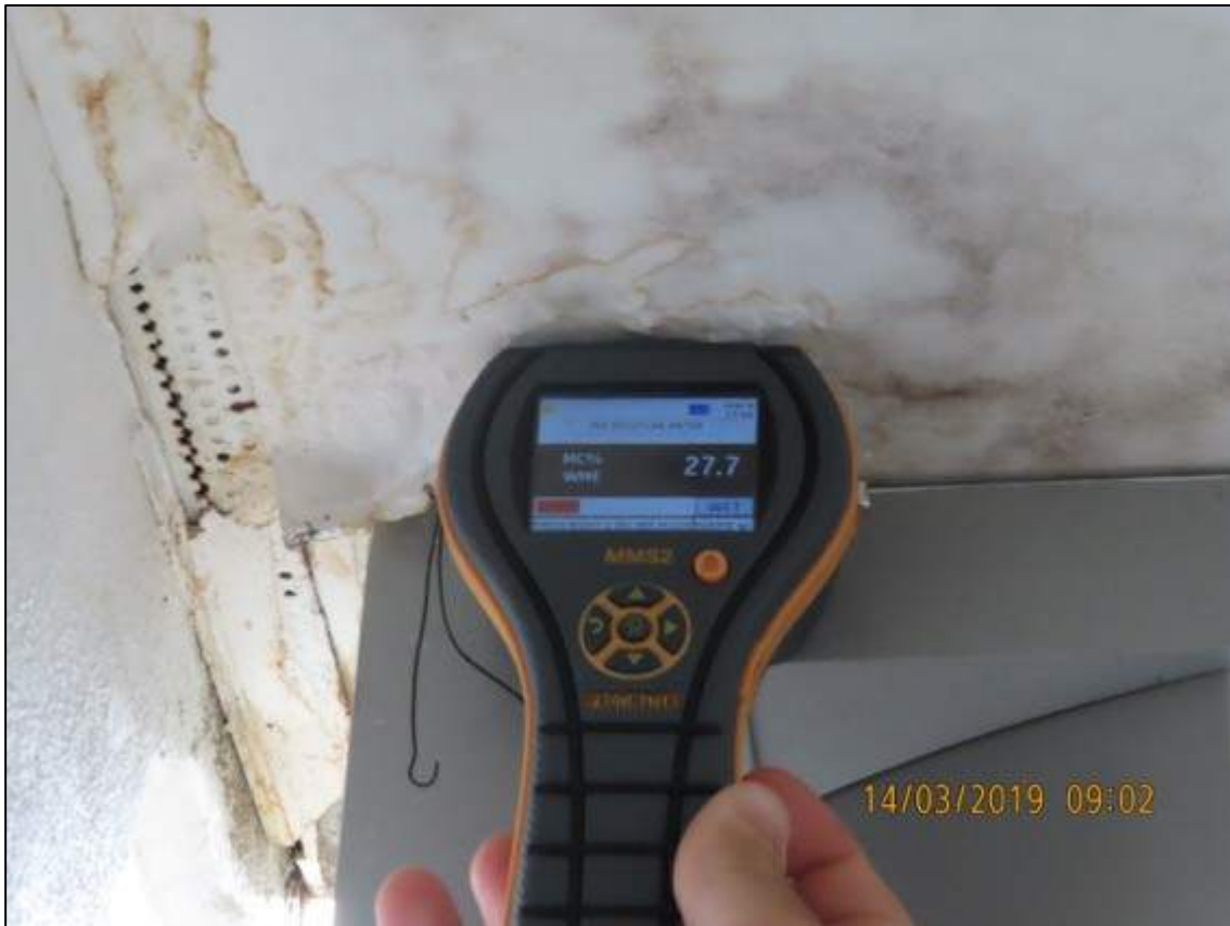
Photograph 50: Showing elevated moisture readings to plasterboard ceiling opposite to Unit 14.
