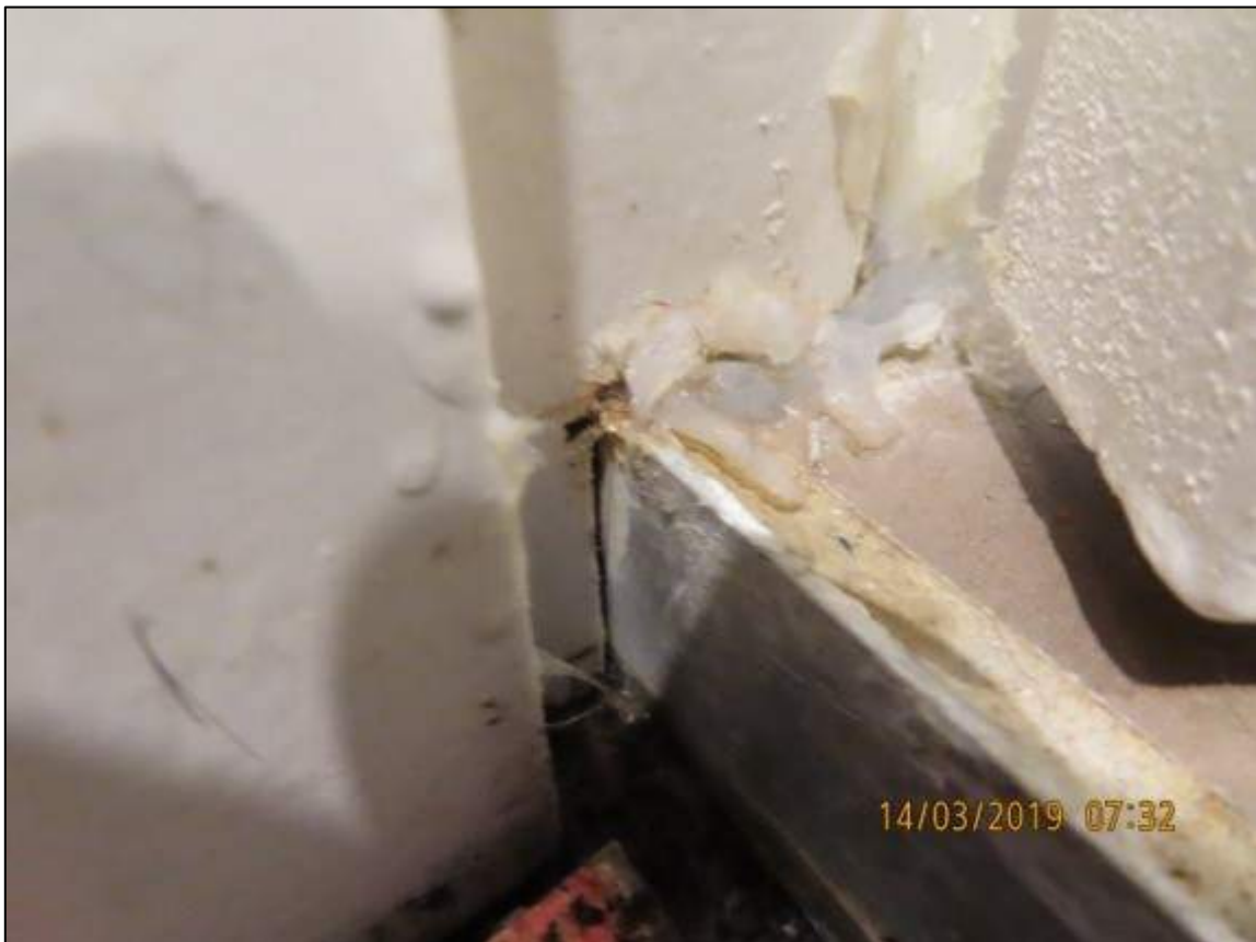
Photograph 4: Showing application of sealant to the threshold of Ensuite in Unit 4.
