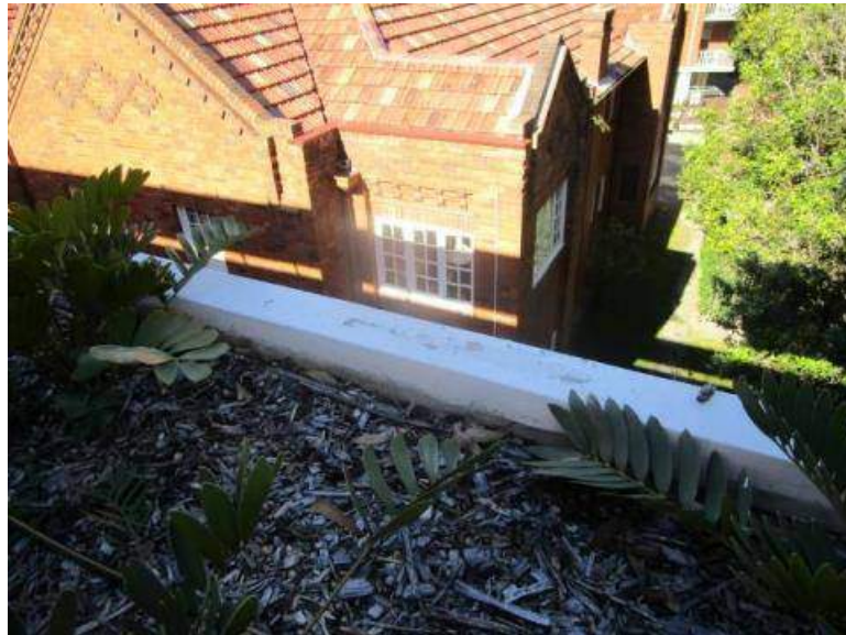
Paintwork to masonry balustrade is deteriorating, recommend rectification.
