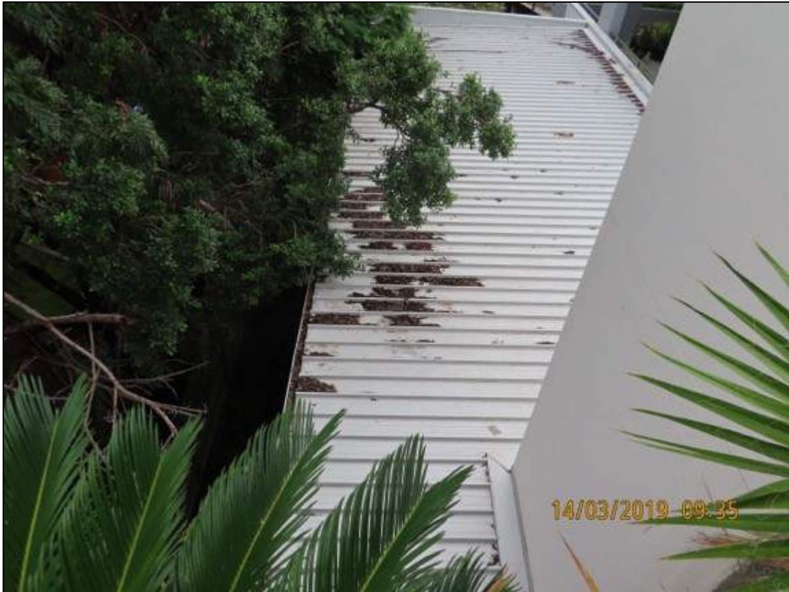
Photograph 56: Showing debris in gutter of aluminium sheeting roof.
