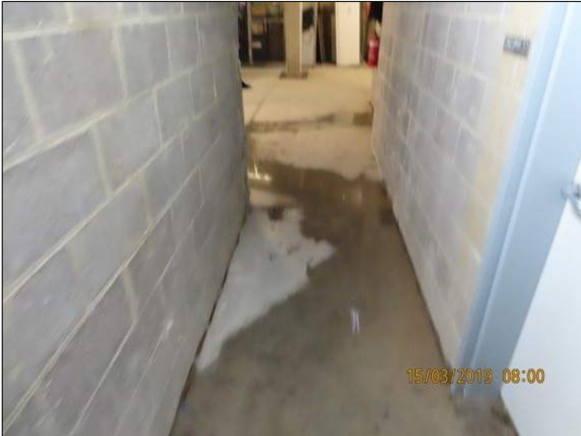
Photograph 58: Showing further view of water ponding opposite northern fire stairs entry of Level 3 basement.
