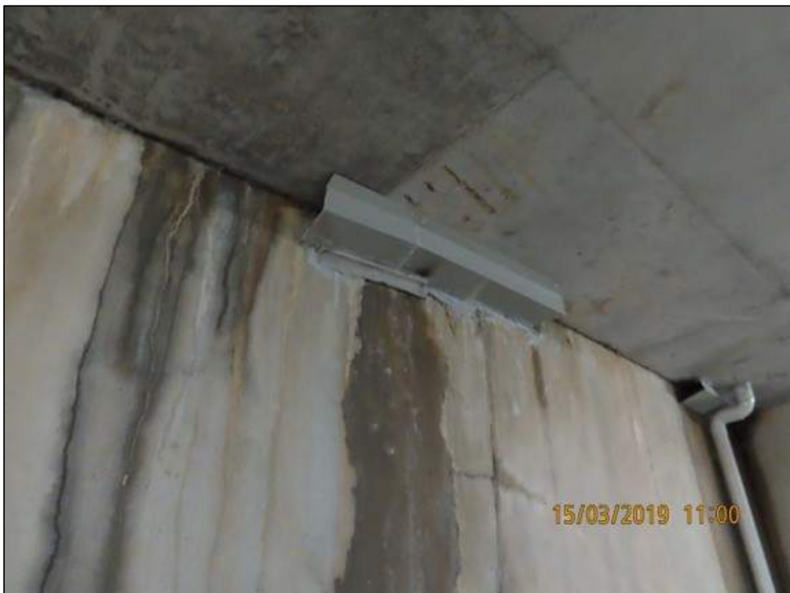
Photograph 65: Showing delamination to drip tray adjacent to car space 1.
