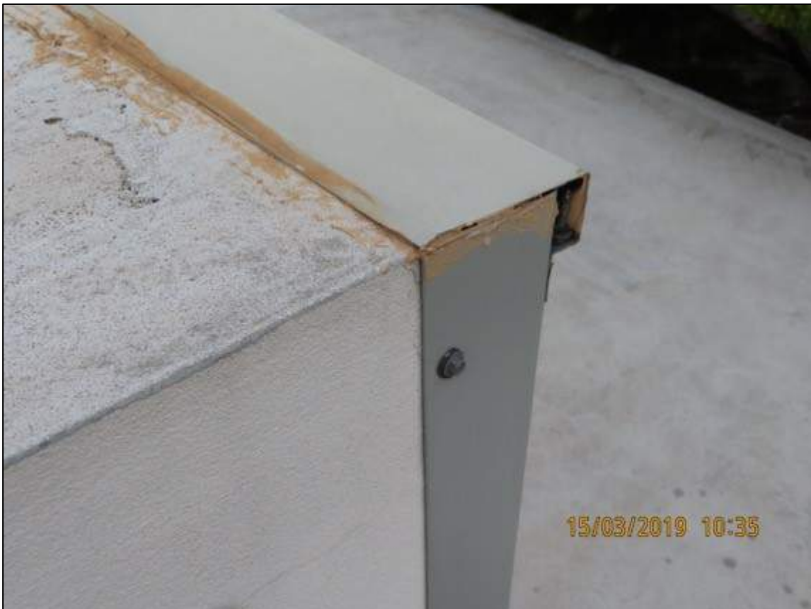
Photograph 71: Showing application of sealant to rooftop perimeter capping.
