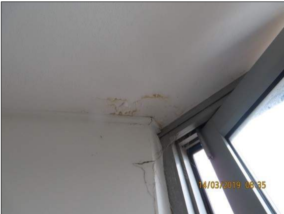
Photograph 15: Showing water damage, staining and blistering plasterboard ceiling adjacent to head of Enclosed balcony windows of Unit 11.
