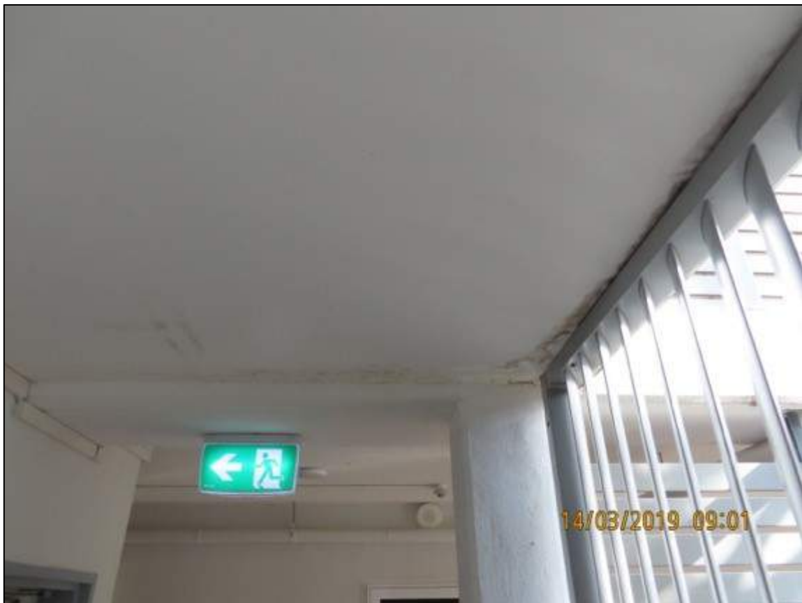
Photograph 48: Showing water staining and blistering plasterboard ceiling opposite to Unit 14.
