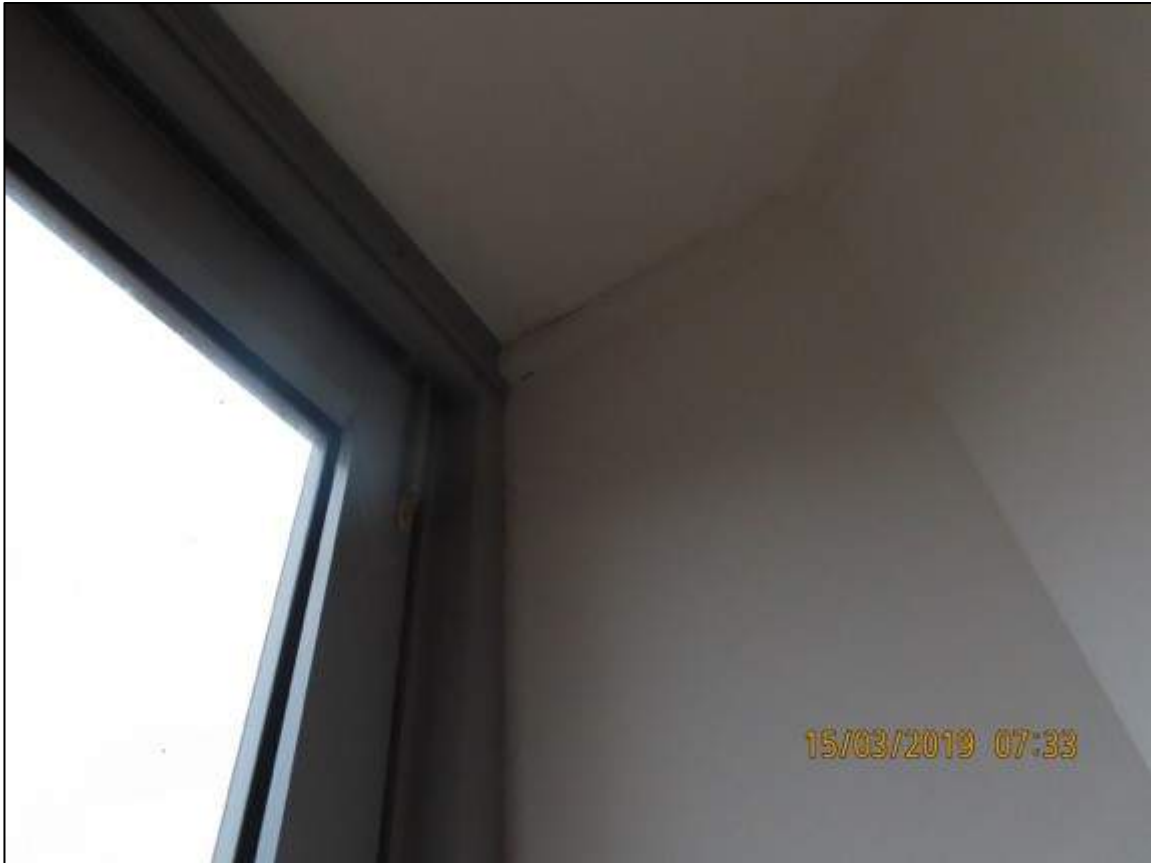
Photograph 24: Showing water staining and damage adjacent to head of Enclosed Balcony windows of Unit 17.
