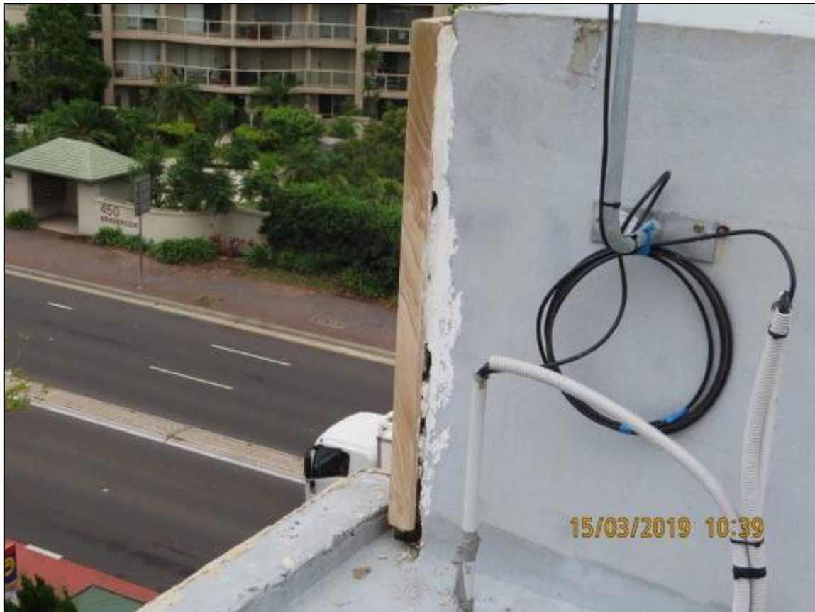
Photograph 78: Showing previous patch repairs to rooftop in form of timber board.
