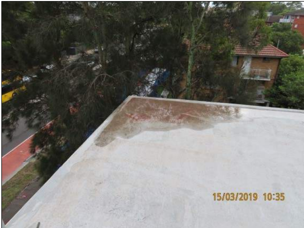
Photograph 68: Showing ponding water to exposed area of rooftop.
