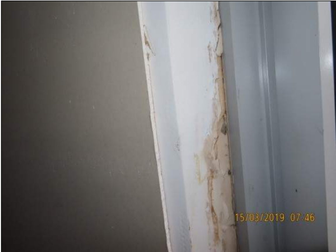
Photograph 26: Showing water damage adjacent to Enclosed Balcony windows of Unit 18.
