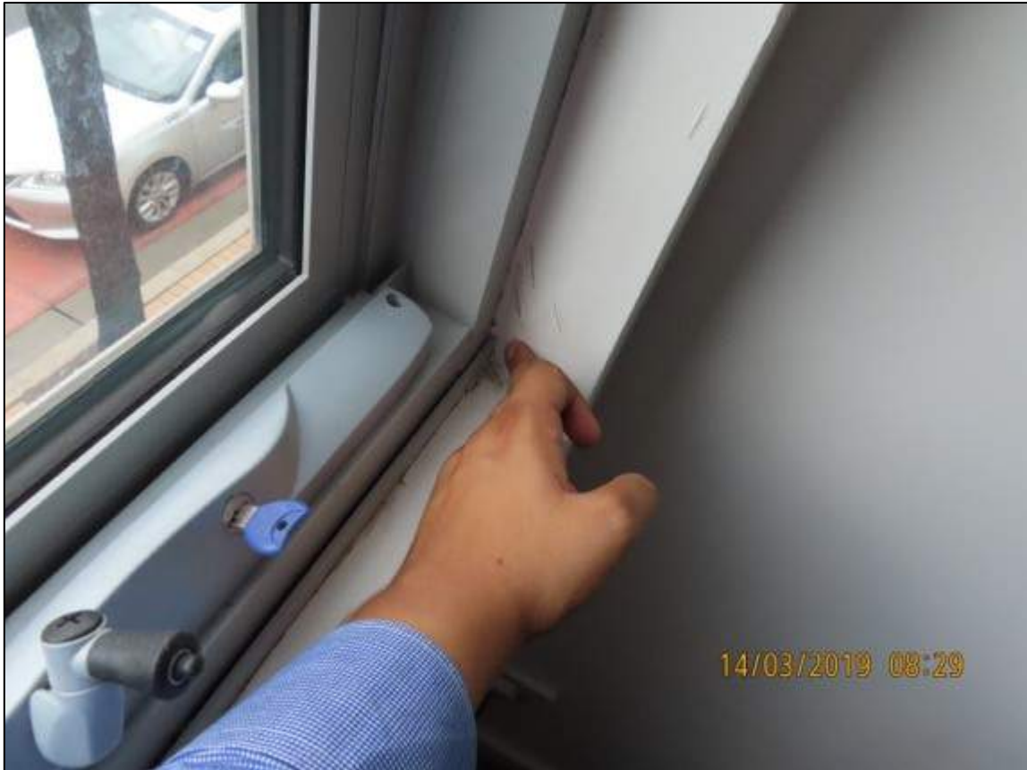
Photograph 12: Showing water damage adjacent to Bedroom window in Unit 8.
