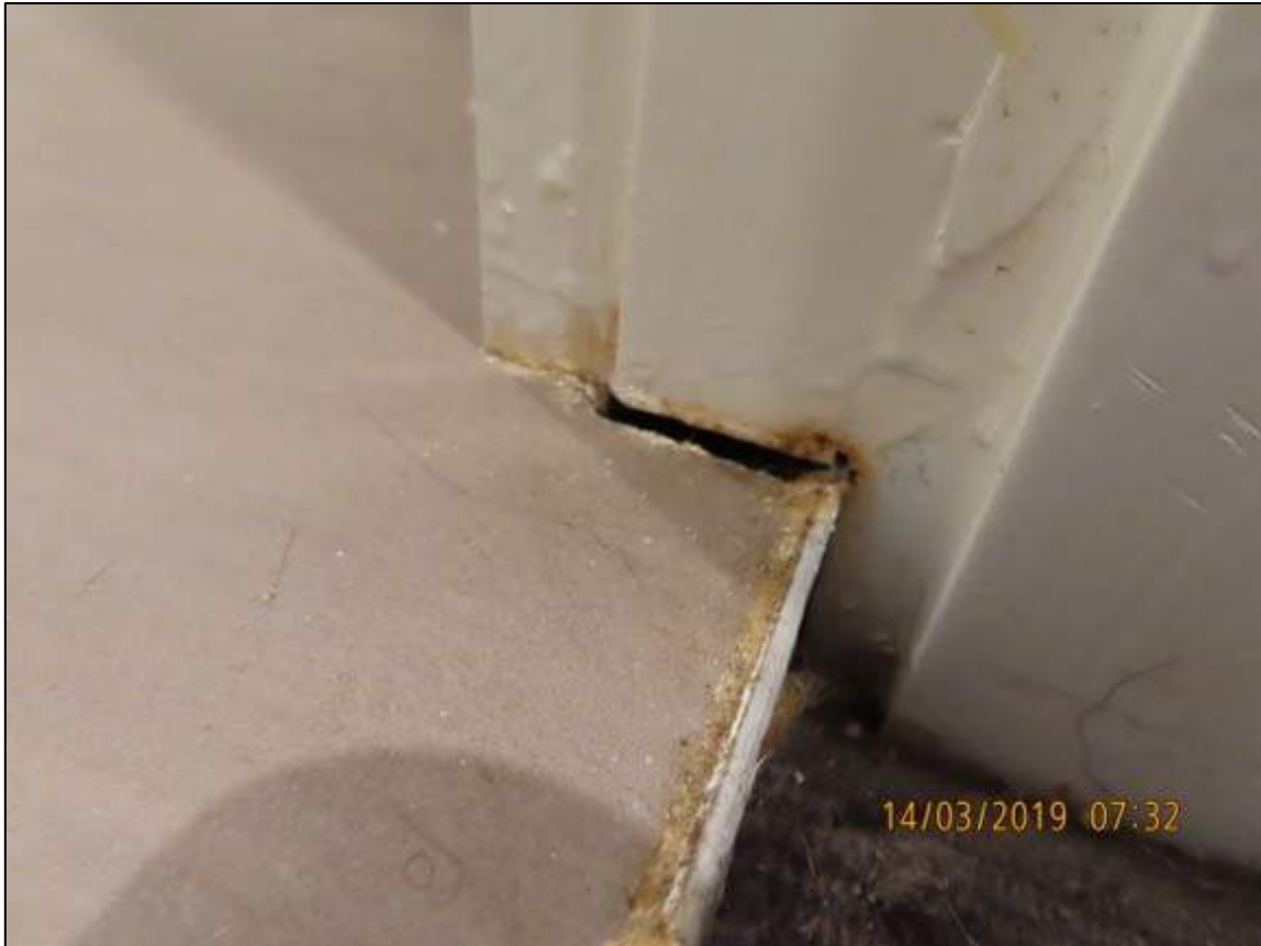
Photograph 3: Showing unsightly gap at threshold of Ensuite in Unit 4.
