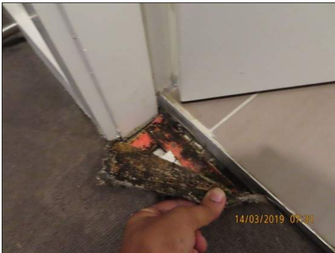
Photograph 2: Showing water staining to the smooth edge of carpet adjacent to threshold of Ensuite of Unit 4.
