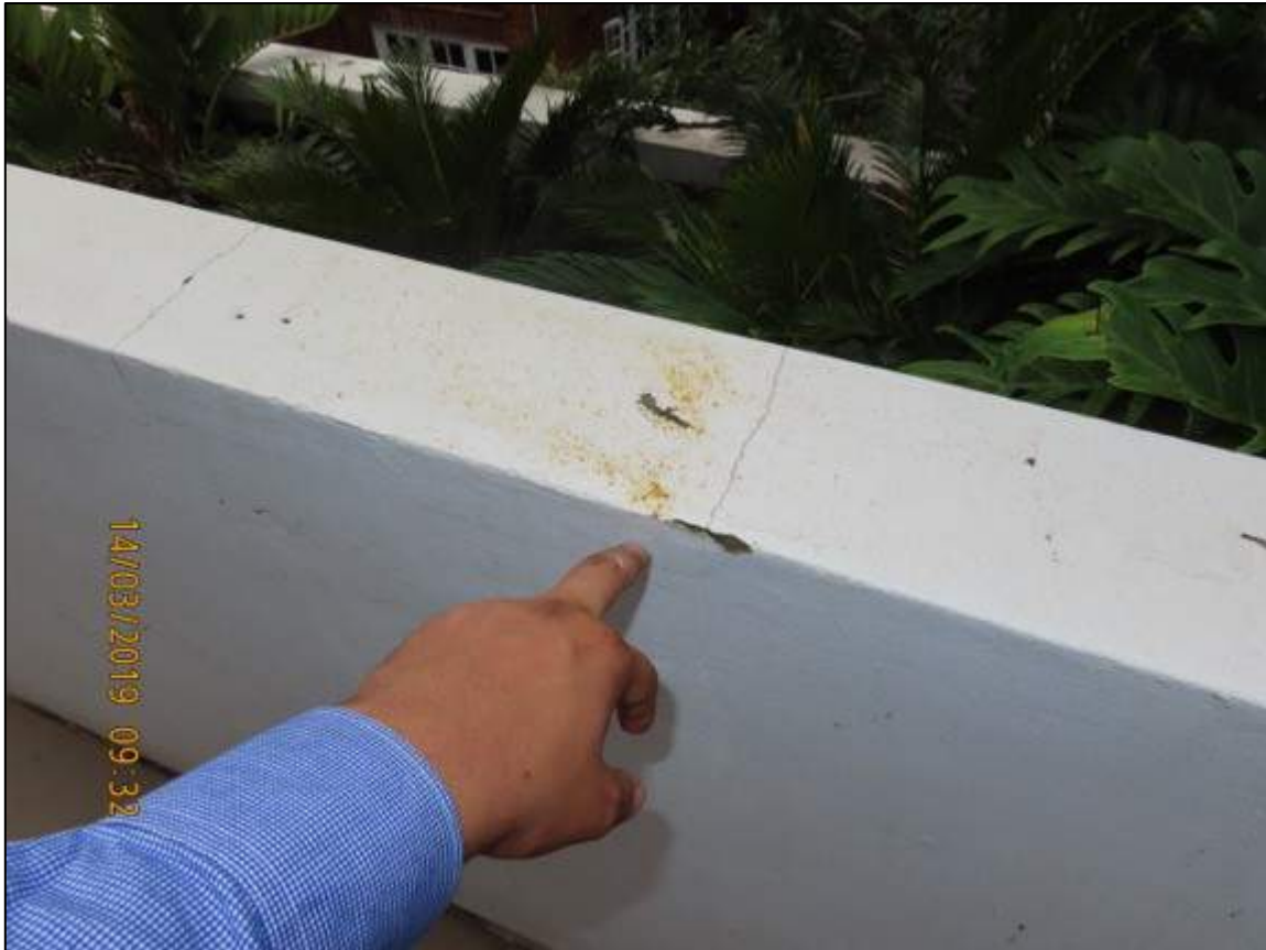
Photograph 54: Showing cracking and corrosion to Level 3 external common area planterboxes.
