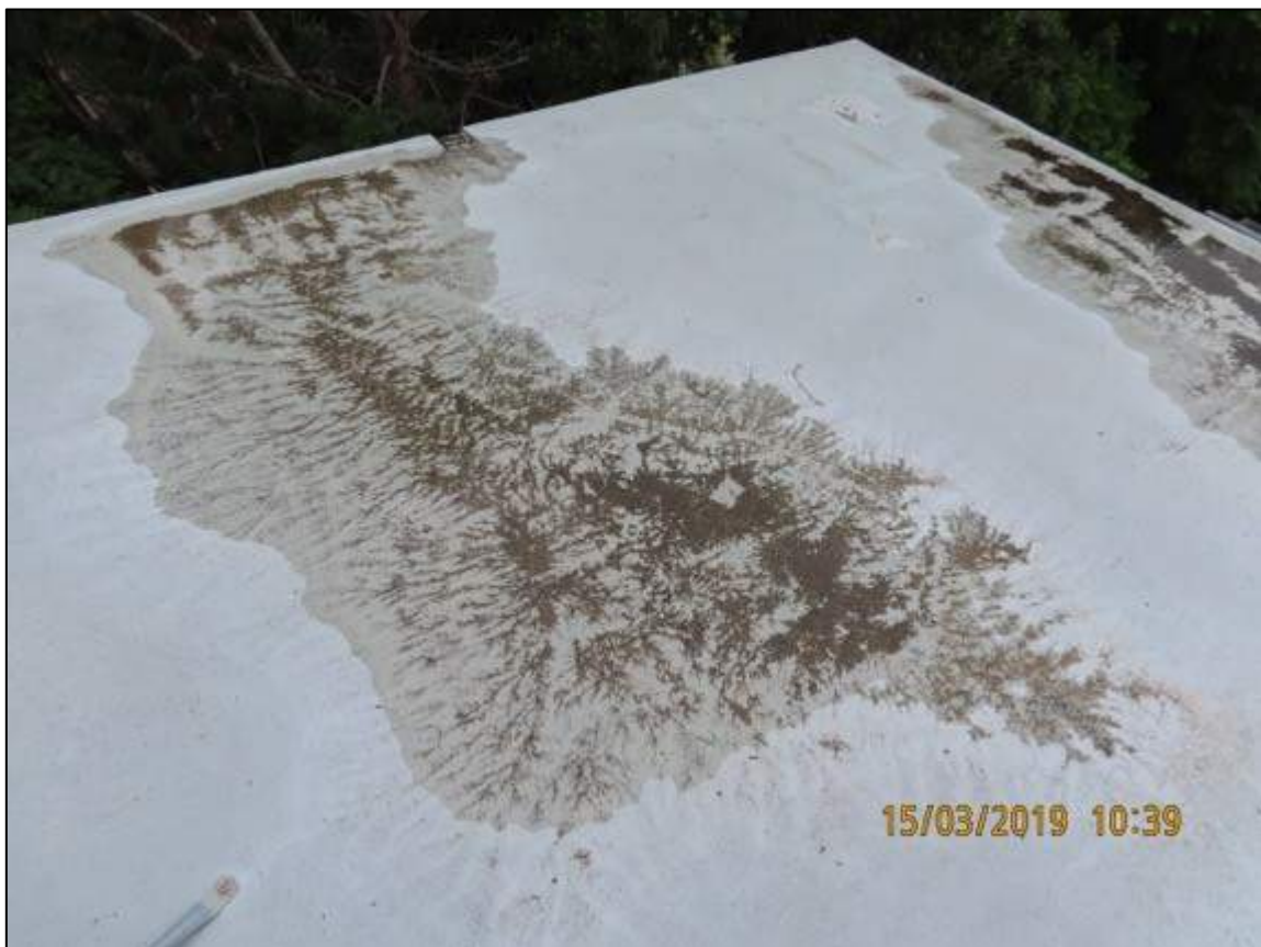
Photograph 79: Showing ponding water to rooftop.
