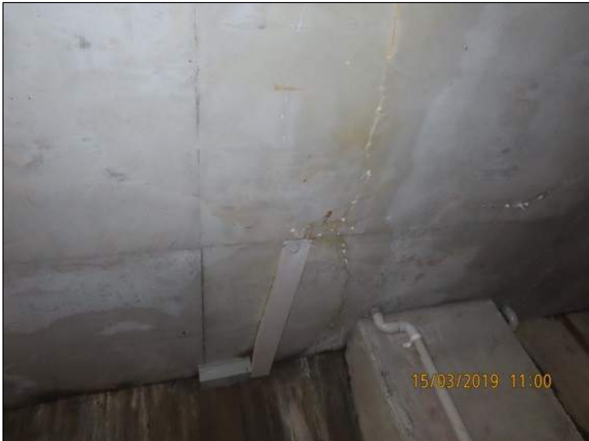
Photograph 64: Showing further view of efflorescence emanating out of cracking of soffit.
