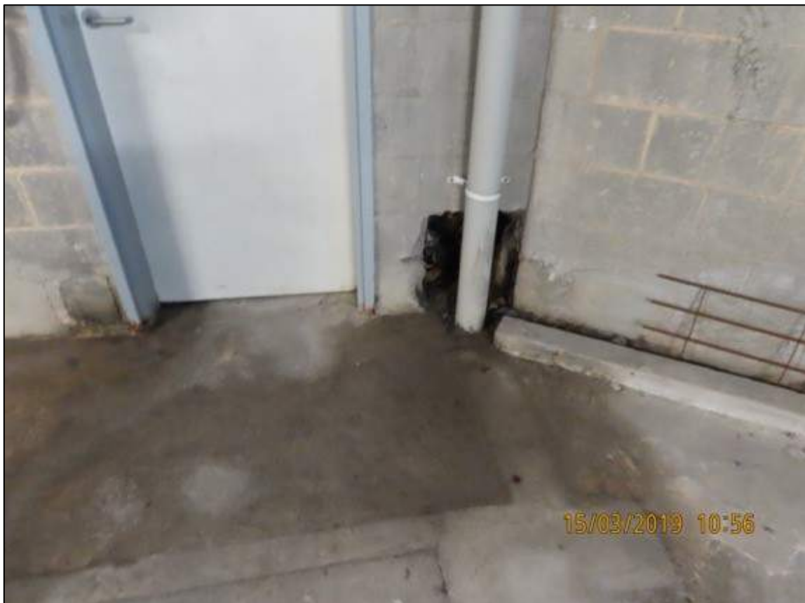
Photograph 59: Showing water ponding and corrosion to entry doors of northern fire stairs on Level 3 basement.
