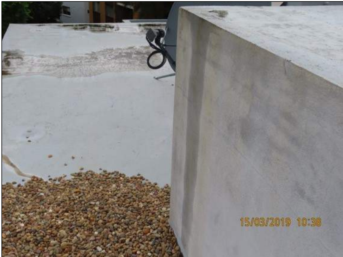
Photograph 76: Showing craze cracking to rooftop façade wall.
