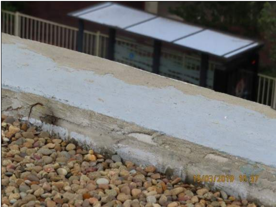
Photograph 74: Showing further view of degradation of waterproofing membrane to perimeter edge.
