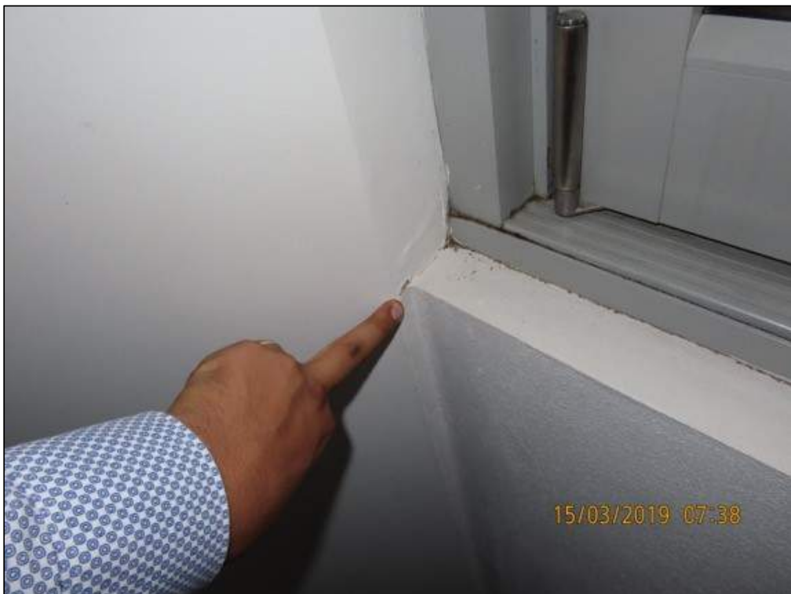
Photograph 33: Showing water damage adjacent to Enclosed Balcony windows of Unit 19.
