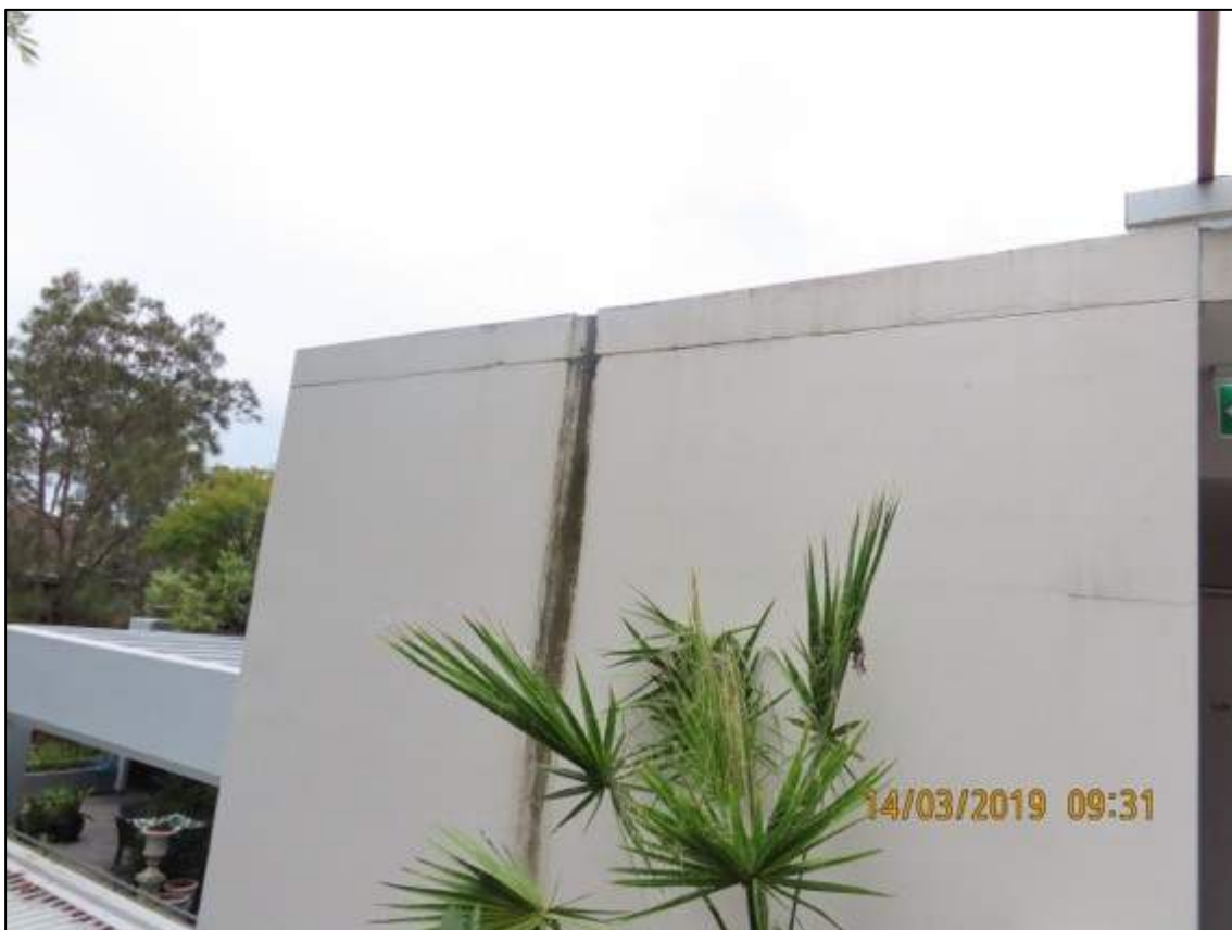
Photograph 51: Showing water staining to facades emanating from rooftop.
