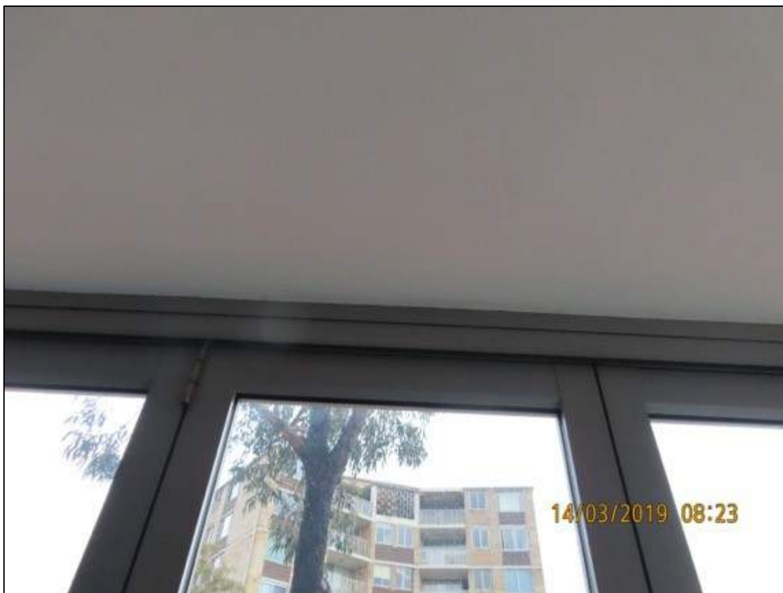
Photograph 10: Showing blistering plasterboard and water staining to head of Enclosed balcony windows in Unit 8.
