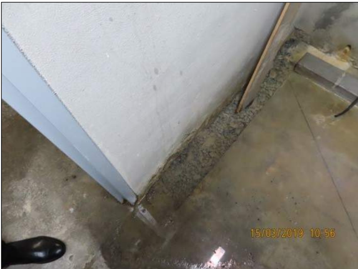
Photograph 61: Showing overflow of water in perimeter hob in northern fire stairs on Level 3 basement.
