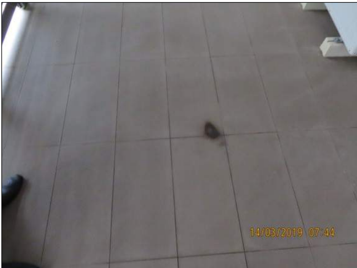
Photograph 47: Showing efflorescence staining to flooring tile of Level 2 internal common area.
