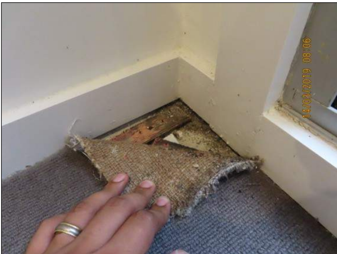
Photograph 6: Showing water staining to smooth edge of carpet adjacent to courtyard sliding door of Bedroom 1 in Unit 5.
