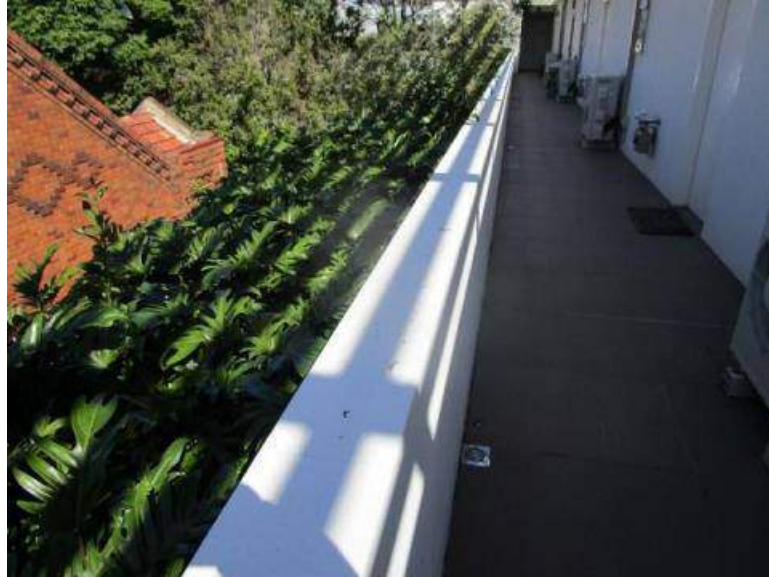
Paintwork to masonry balustrade is deteriorating, recommend rectification.
