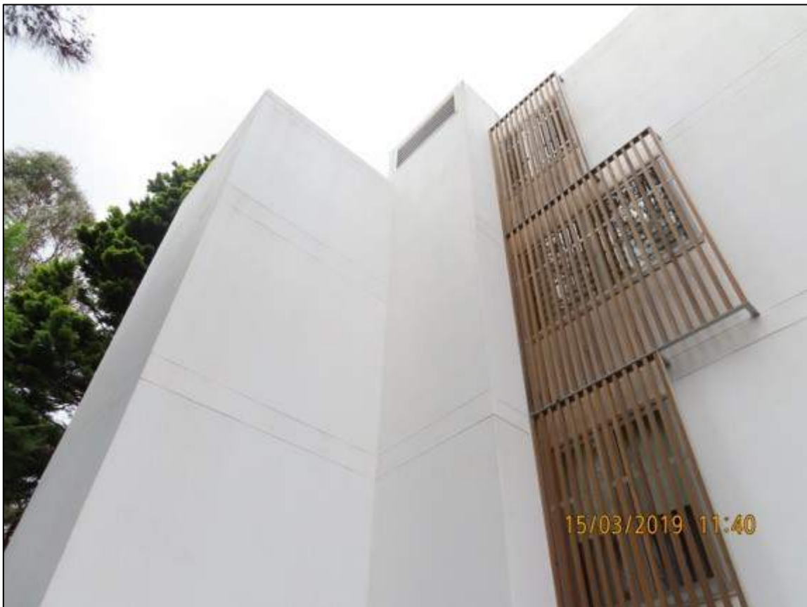
Photograph 67: Showing absence of movement joints to the façade on the eastern elevation.
