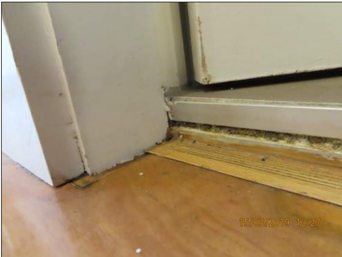
Photograph 39: Showing waterproofing detailing where new flooring tiles are placed above original tiles of Bathroom of Unit 22.
