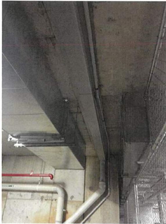
Photo 5: Sheet metal catch drain fitted to construction joint between the ground floor slabs of buildings A and B on B1. This drain was found to be leaking.
