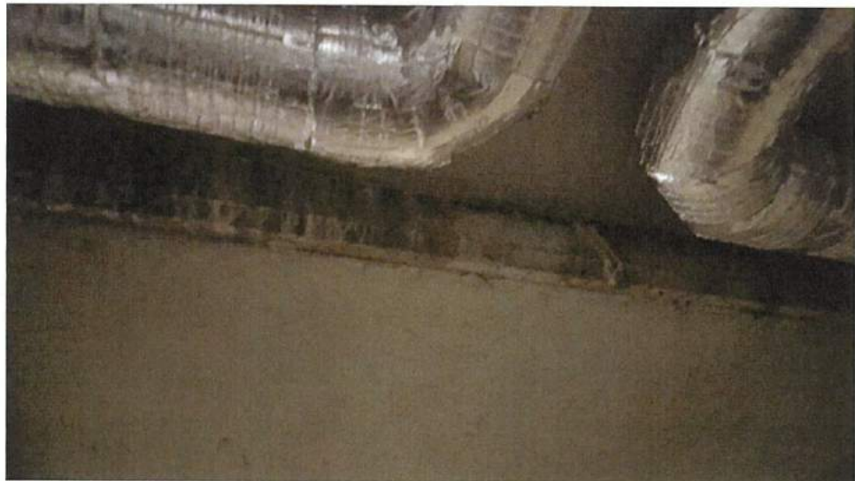
Photo 4: Leak at cold joint between floor slab and south side of elevator structure.
