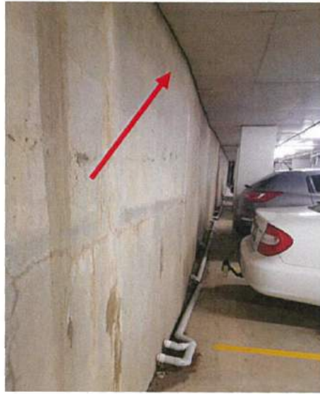
Photo 1: Photo showing a significant bow in the boundary wall on B3.
