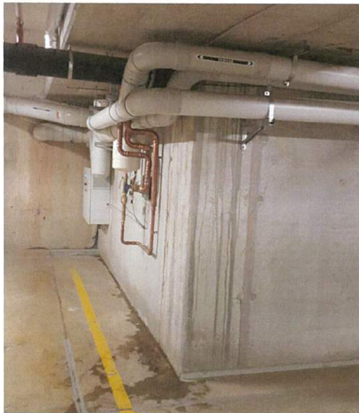
Photo 2: Leak at storm water drainage line entry point to retention tank on B1.
