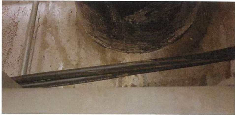
Photo 3: Closer view of the leaking junction between the cast iron pipe and concrete wall of the retention tank, this is a close up of the leak shown in Photo 2 above.
