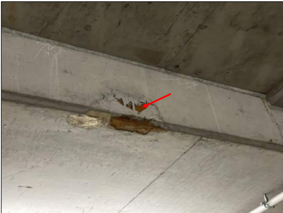
Photograph 4: Leftover formwork in the concrete slab in the carpark
