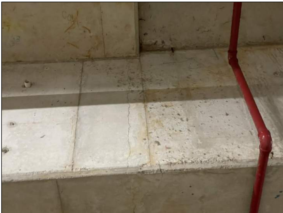
Photograph 6: Crack to the concrete beam in the carpark
