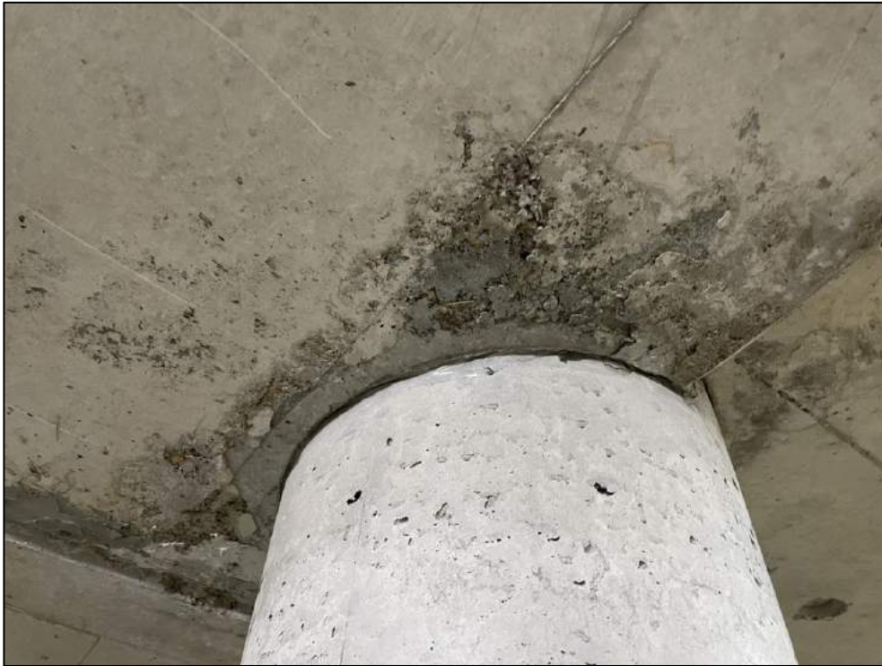
Photograph 5: Concrete honeycombing on the carpark slab soffit around the column
