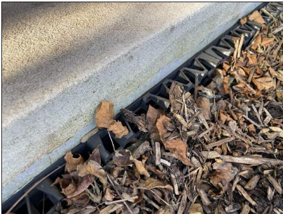
Photograph 7: Waterproofing membrane cracking and not up and over the plant box wall in the common courtyard
