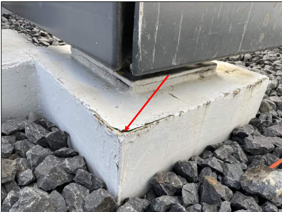
Photograph 2: Delaminated waterproofing membrane on the concrete plinth edges (10 Burroway Rd.)
